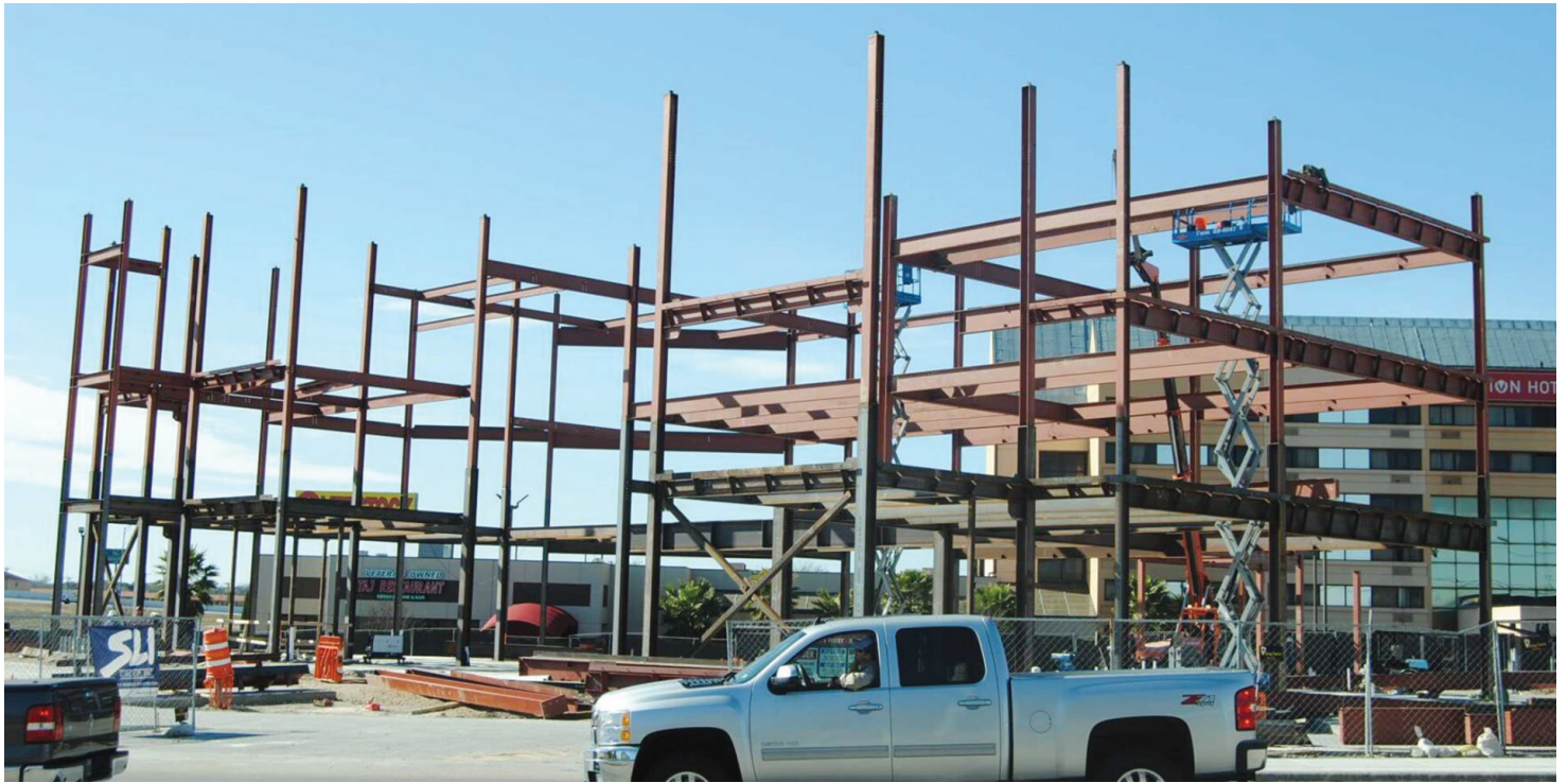
Progress continues on the new Killeen corporate headquarters for First National Bank Texas.
