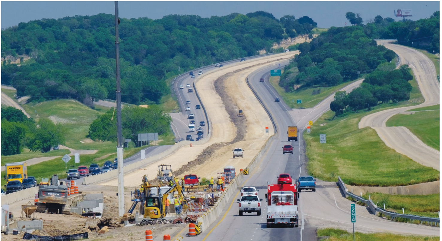
Lane widening projects continue between Harker Heights and Belton on Interstate 14. Phase 2 should wrap up later this year, weather permitting.
