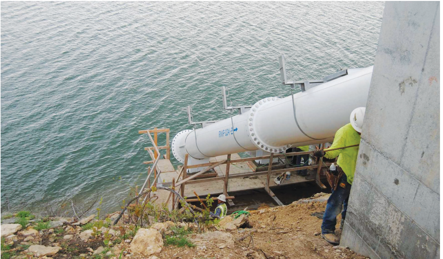
Intake pipes move down the cliff toward Stillhouse Hollow Lake and will be lowered to pull water from the lake at the new water treatment plant.
