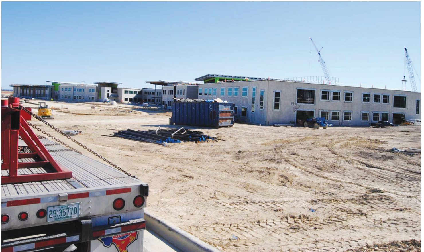
Construction of Killeen ISD's Chaparral High School is underway. The district's sixth high school is set to open in the fall of 2022.
