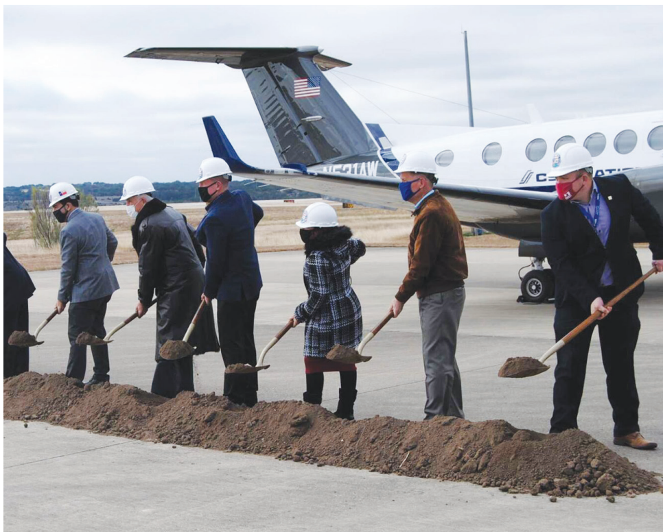
Local officials and project members pick up dirt in their shovels to signify the groundbreaking of the new hangar at the Killeen-Fort Hood Regional Airport in December.
