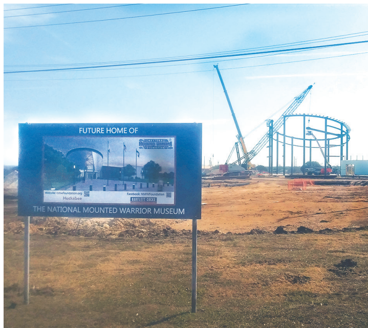
Construction is underway on the Mounted Warrior Museum at Fort Hood.
