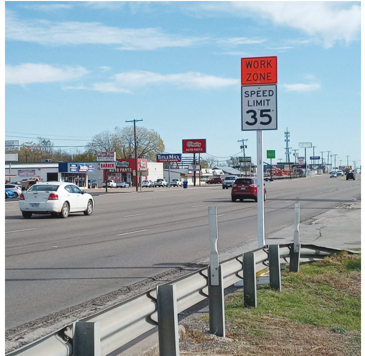
The speed limit has been lowered to 35 mph along part of Business Highway 190 in Copperas Cove while crews work to add a sidewalk.
