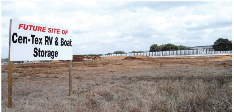
Construction is underway for Cen-Tex RV and Boat Storage near Paddy Hamilton Road in Nolanville.
