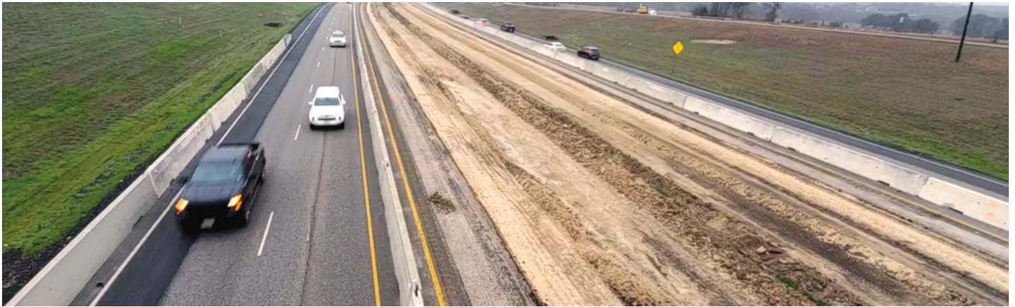
Motorists drive through a construction zone on Interstate 14 in Nolanville.
