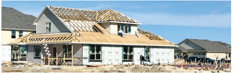
New homes are under construction on Achille Drive in Harker Heights.
