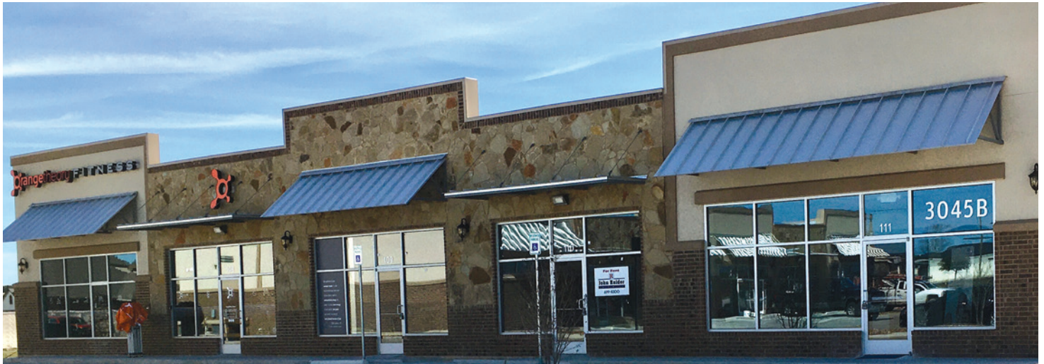
Construction is underway on a new strip mall in Harker Heights to make room for more businesses.
