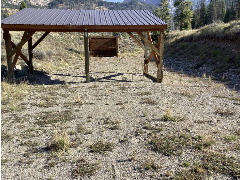
Photo 3. View of existing shooting infrastructure on the northern end of the Property (10/3/2024). Existing structures will be removed and this area will be re-graded with more natural slopes and reclaimed with native grasses and used for shooting sports.
