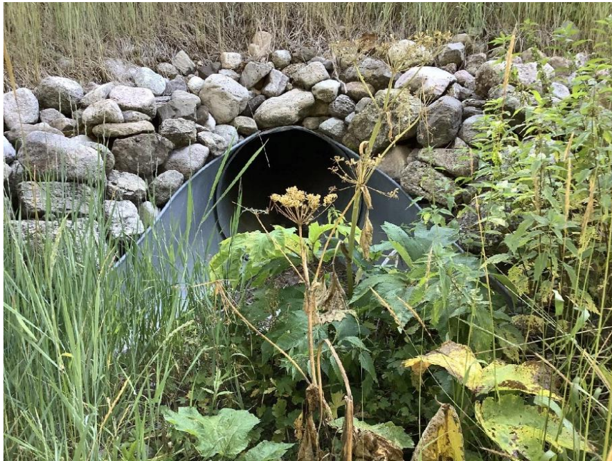
Photo 10 (9/5/2024) - Looking west from within the emergent wetland swale (W1). This culvert provides connectivity between the two segments of the wetland swale. Further downgradient to the west, this swale lacks connectivity with Granite Creek where it appears there was historic connectivity. This disconnection is a result of previous development of a driveway within the Property.
