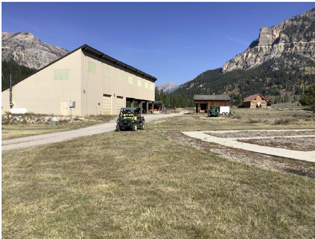
Photo 1. View of the existing shop on the western edge of the Property that will be removed and reclaimed with native vegetation (10/3/2024).
