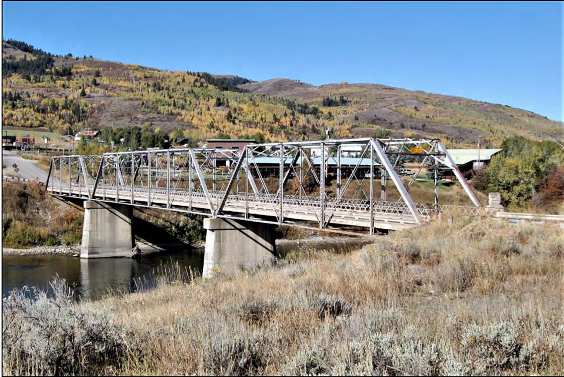
Figure 8. South side of Structure DEY, view to west. (Photo by Rosenbergs, 10/3/2019)
