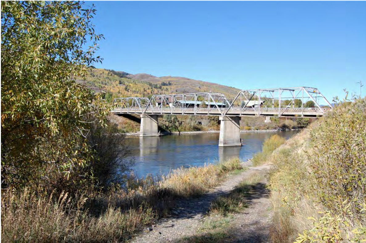
Figure 1: Structure DEY (48TE973) view to west (Rosenberg 2019).
