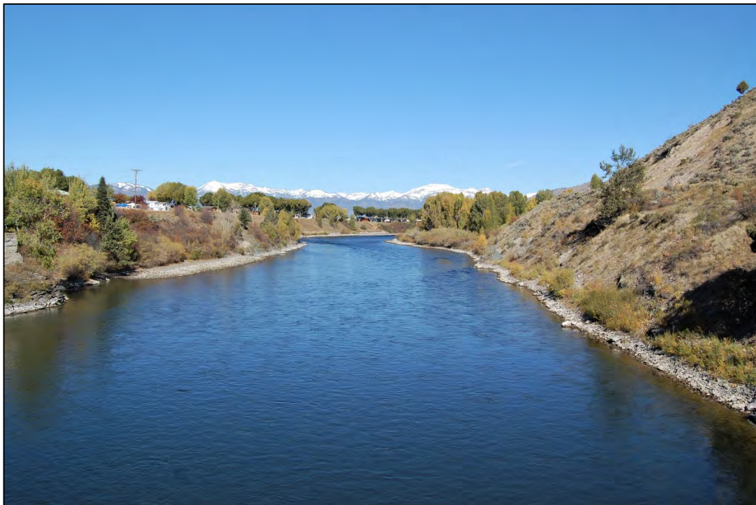
Figure 14. Upstream from bridge, view to north-northwest. (Photo by Rosenbergs, 10/3/2019)
