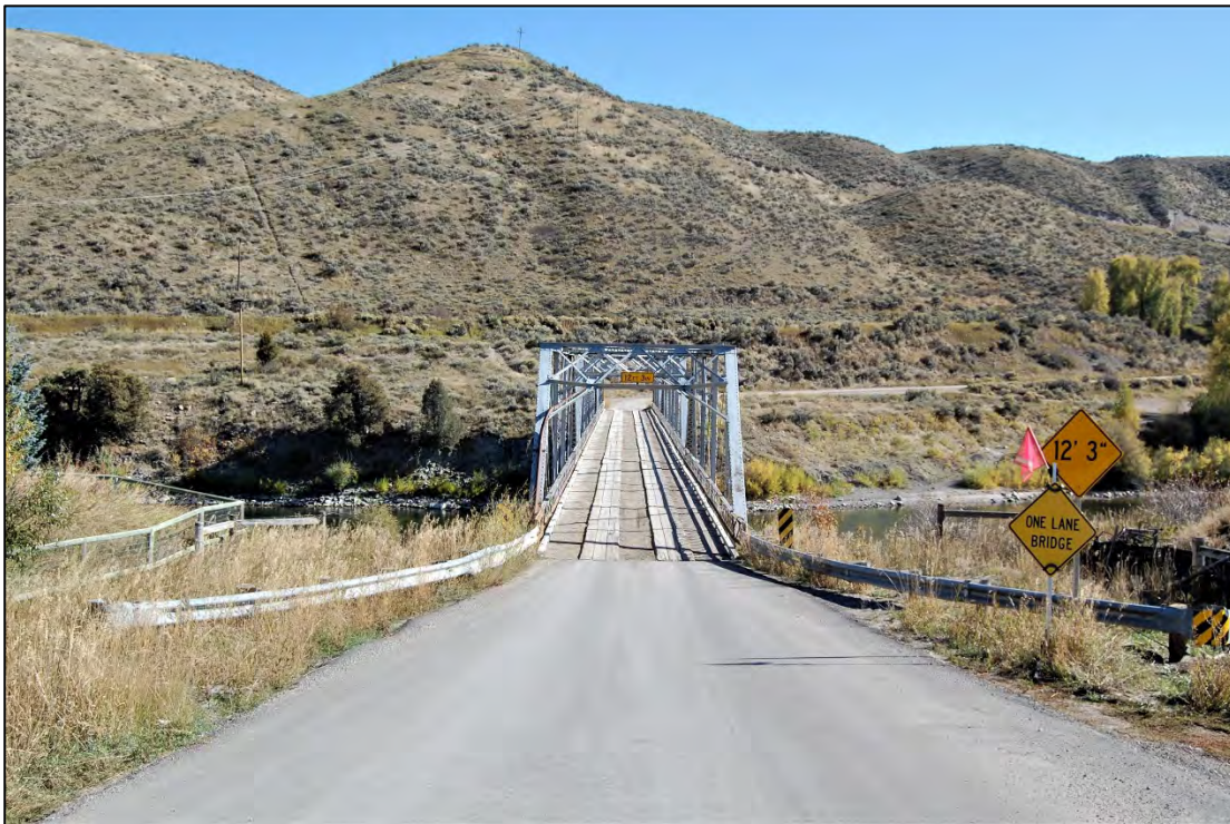
Figure 3. Overview of Structure DEY, which crosses the Snake River about 4 miles north of Hoback Junction on Teton County Road 11. View to east-northeast.
