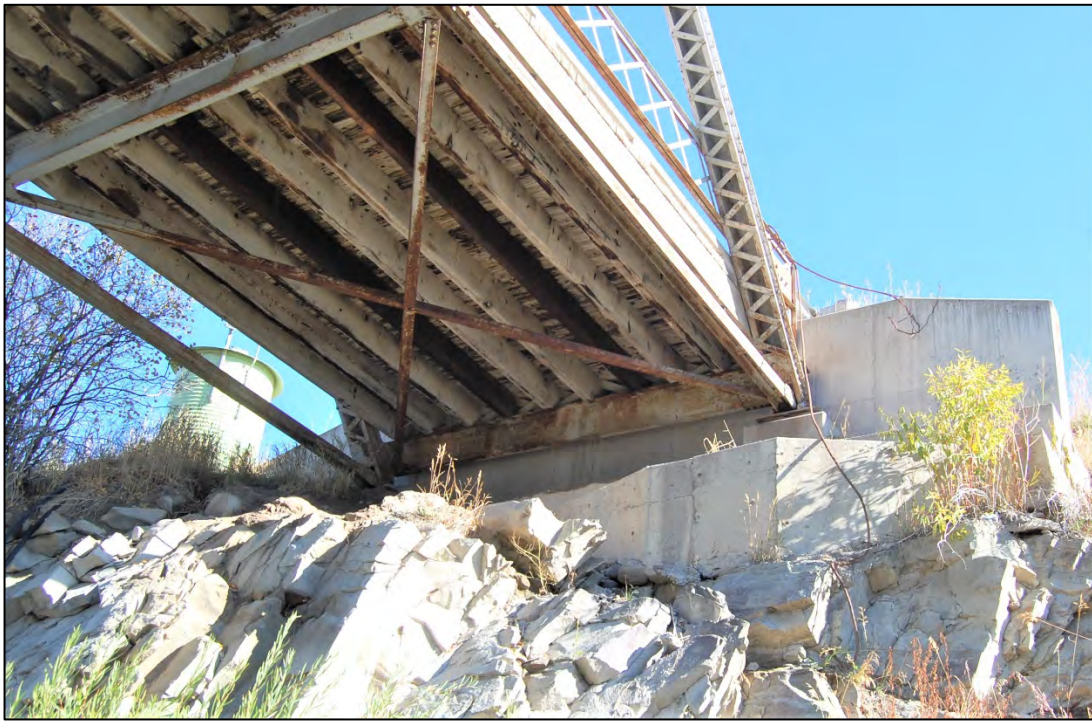
Figure 13. Underside of east end of bridge and the east abutments. (Photo by Rosenbergs, 10/3/2019)
