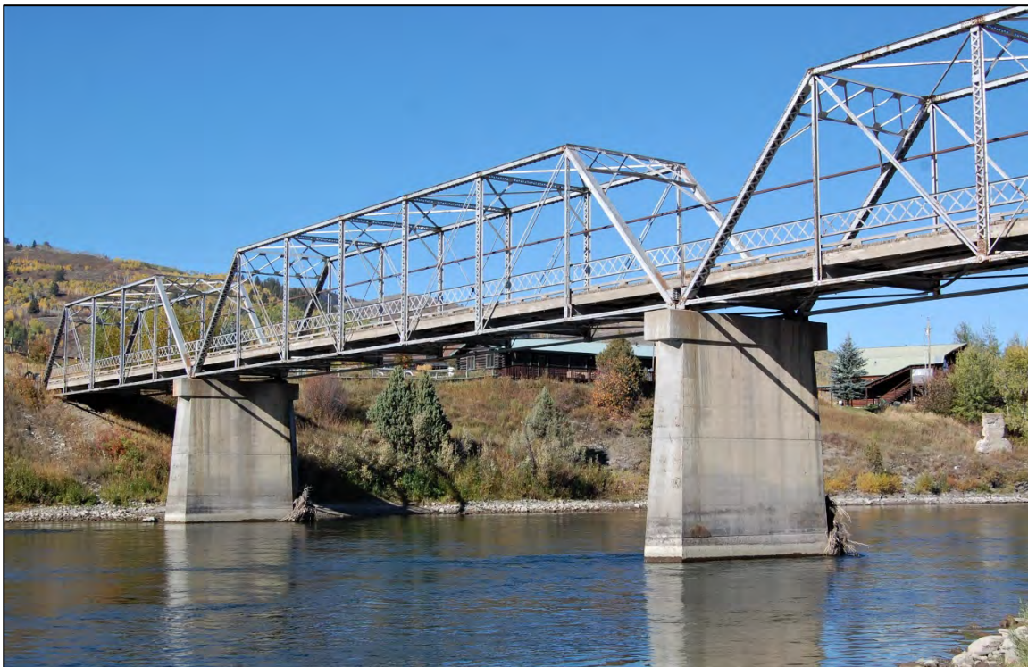
Figure 9. Close up of piers and trusses, view to west. (Photo by Rosenbergs, 10/3/2019)
