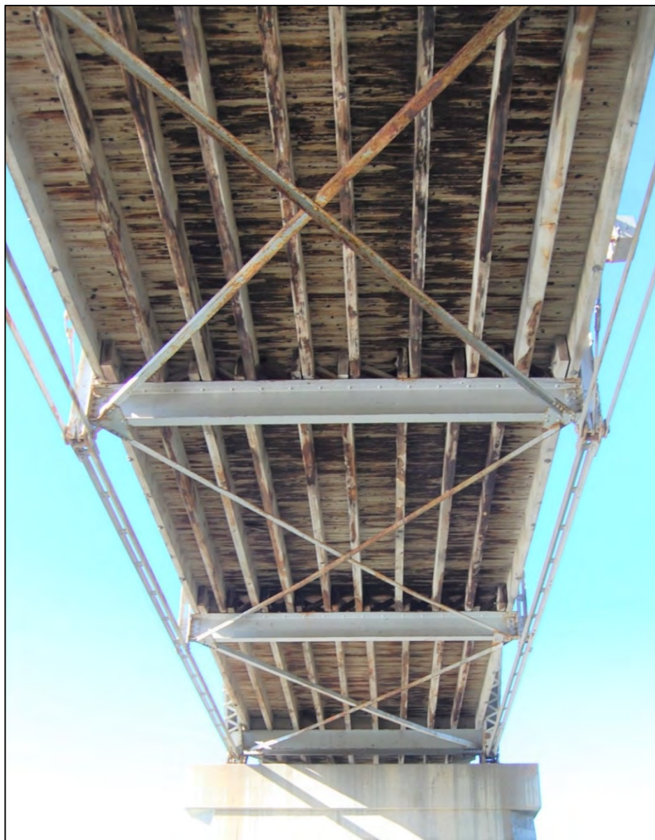
Figure 12. Underside of wood deck with wooden stringers and steel floor beams. (Photo by Rosenbergs, 10/3/2019)
