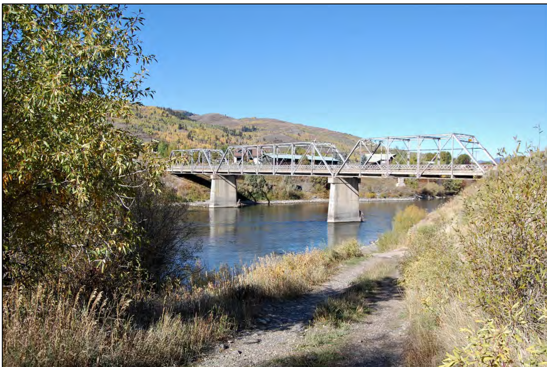
Figure 5. View to west-northwest
