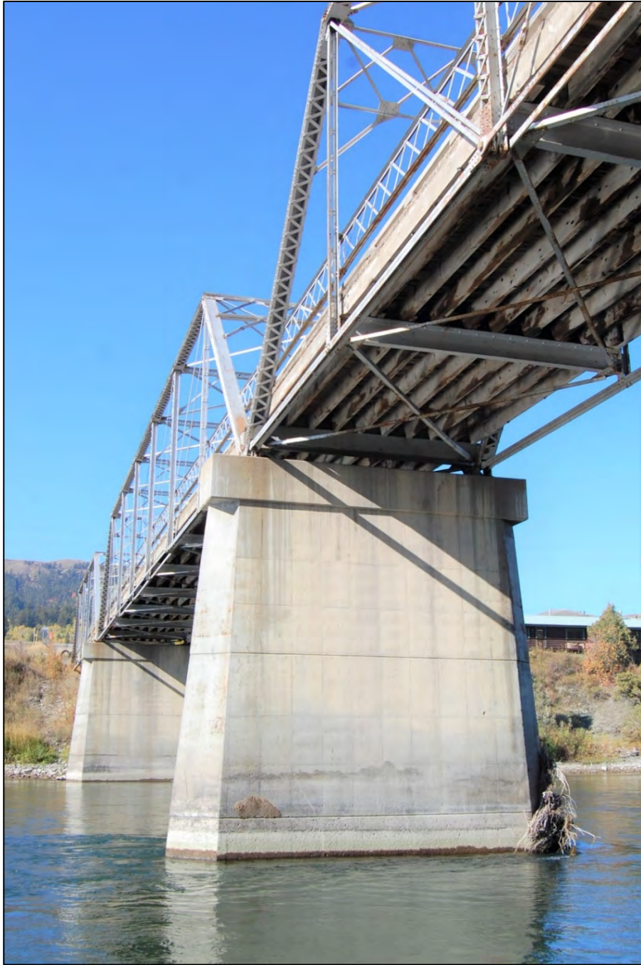
Figure 11. Detail of pier and underside of bridge, view to west. (Photo by Rosenbergs, 10/3/2019)
