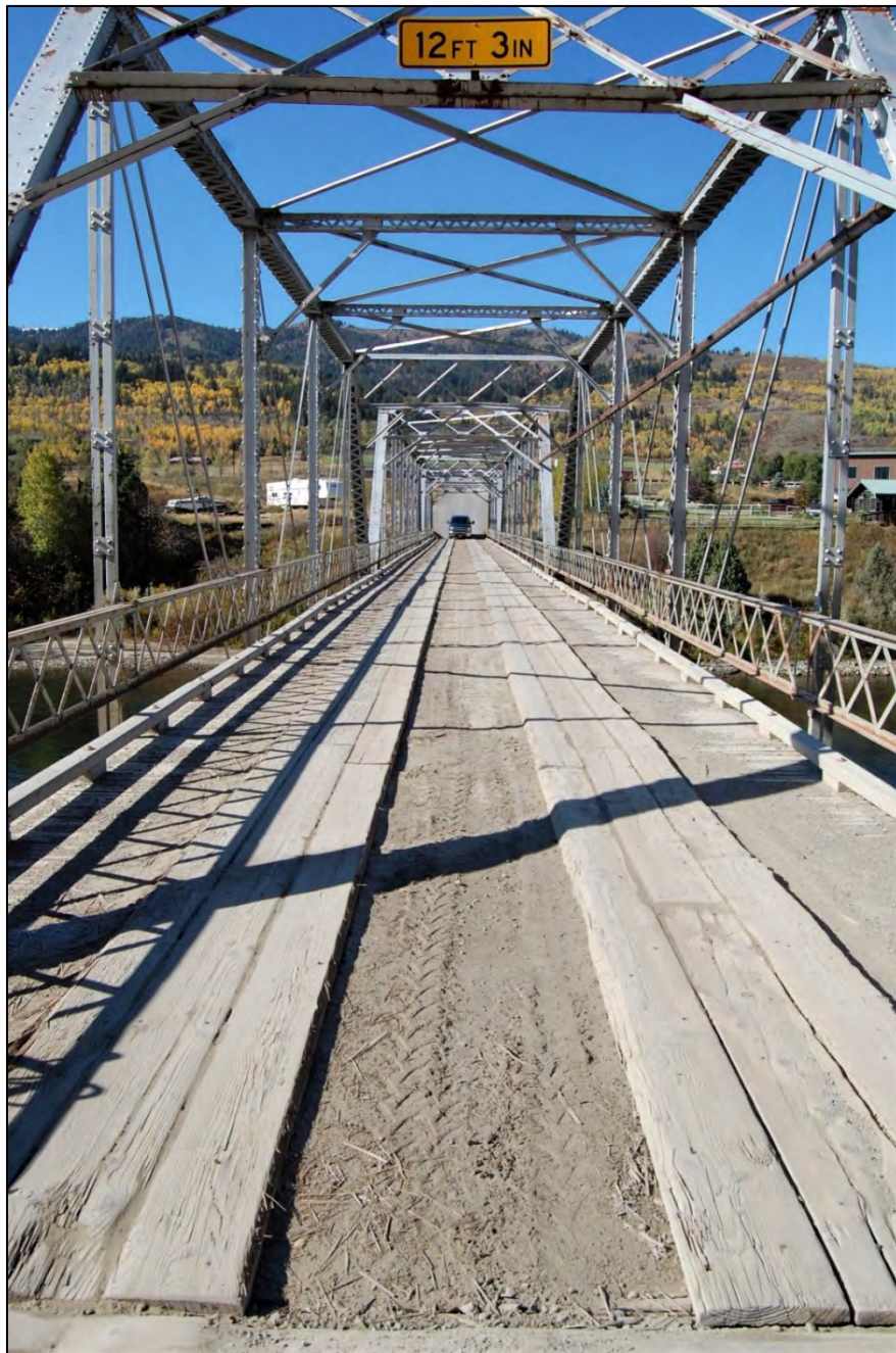
Figure 10. Bridge deck, view to west-southwest. (Photo by Rosenbergs, 10/3/2019)
