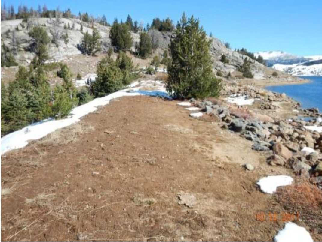
Photo 1. Embankment crest – mature trees on crest and slope.
