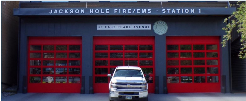
Figure 26: Jackson Hole Fire/EMS Station 1
