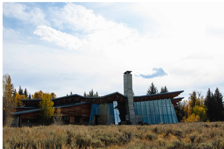
VISITOR CENTER-BUILDING A, D
