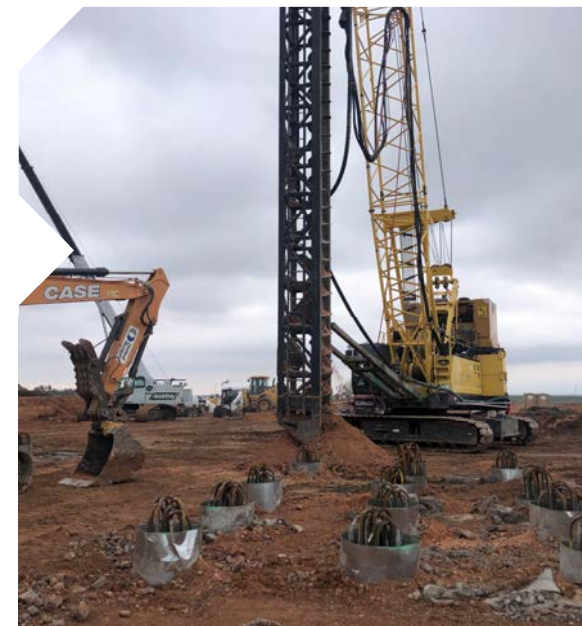
Warehouse Support (Lubbock, Texas) (349) 24in. CFA to 50ft Cobble Obstructions
