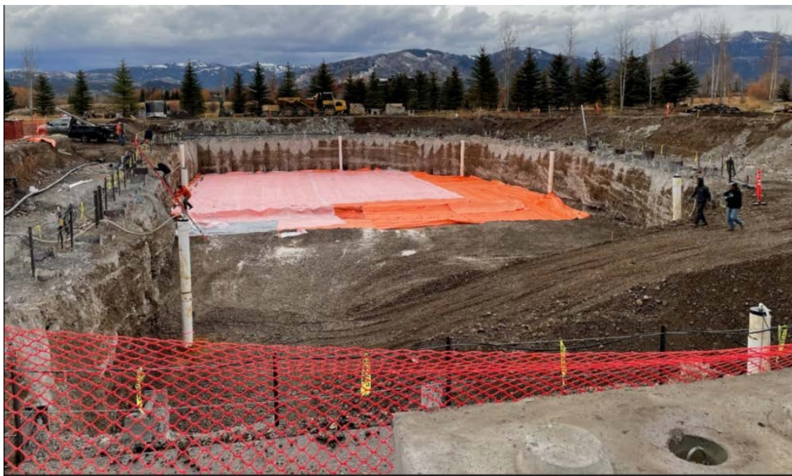
Figure 1: DSM secant pile wall and dewatering system. Teton County, WY (2020)
