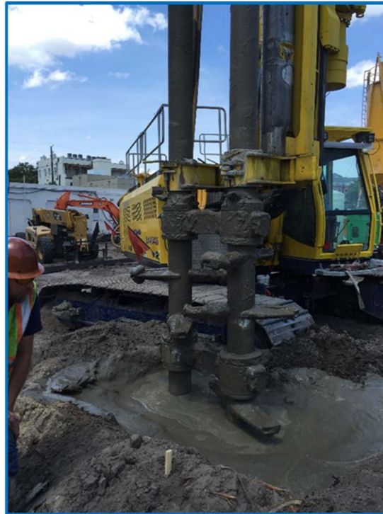
Deep Soil Mixing
