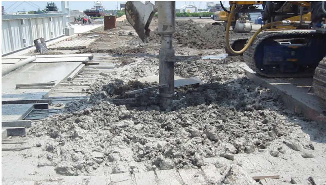
Deep Soil Mixing
