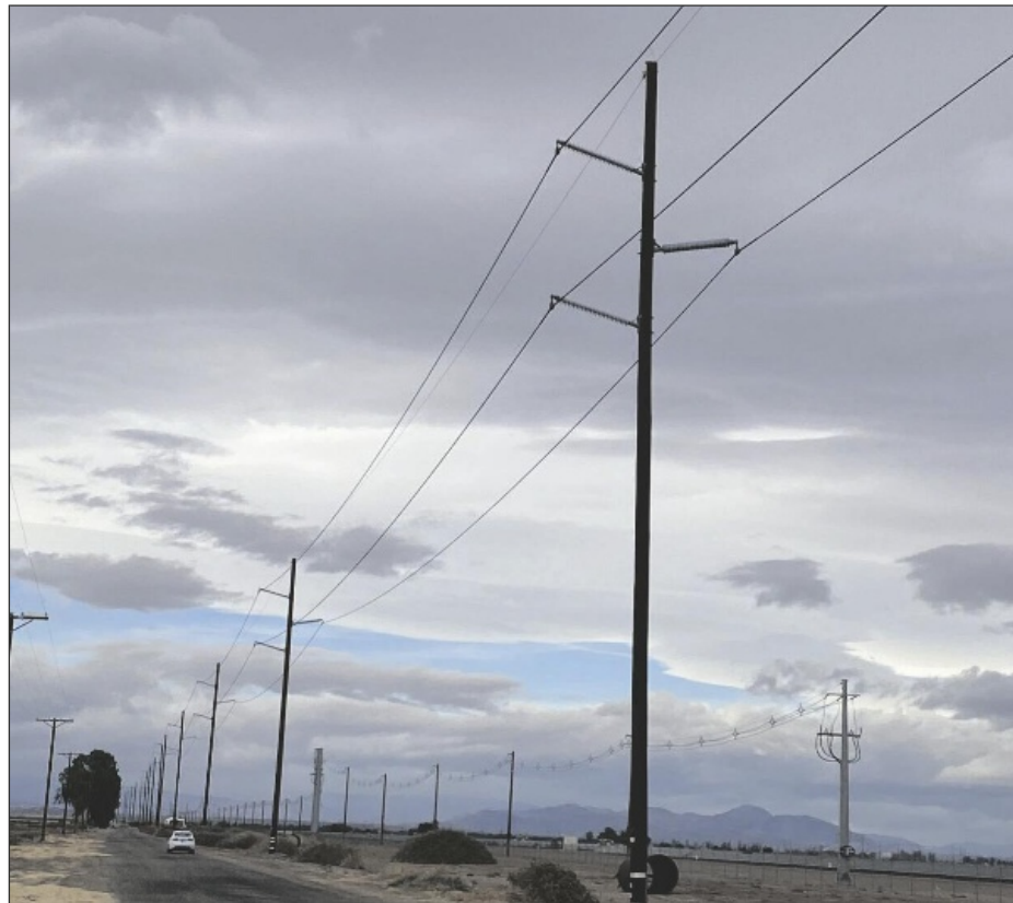
These wooden power poles south of Seeley owned by the Imperial Irrigation District will soon be replaced by steel ones in a $55 million upgrade.
