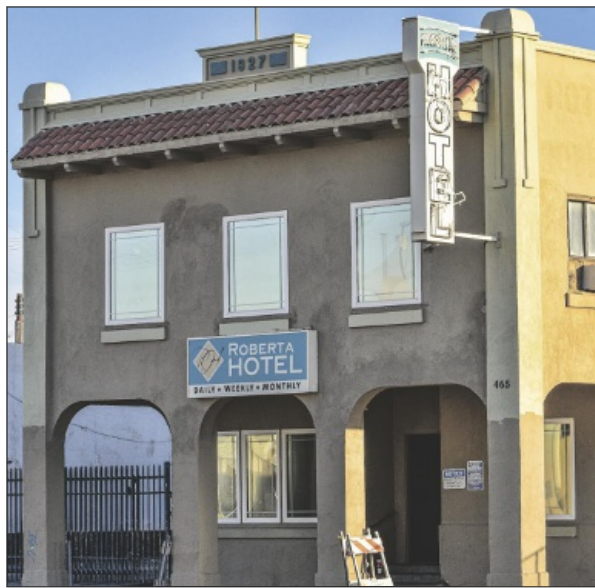
The Roberta Hotel, 465 W. State St., El Centro, as seen on Nov. 16. Tenants there were cleared out Nov. 18 due to the building being red-tagged by the city for safety violations. IVP FILE PHOTO/CORISSA IBARRA
