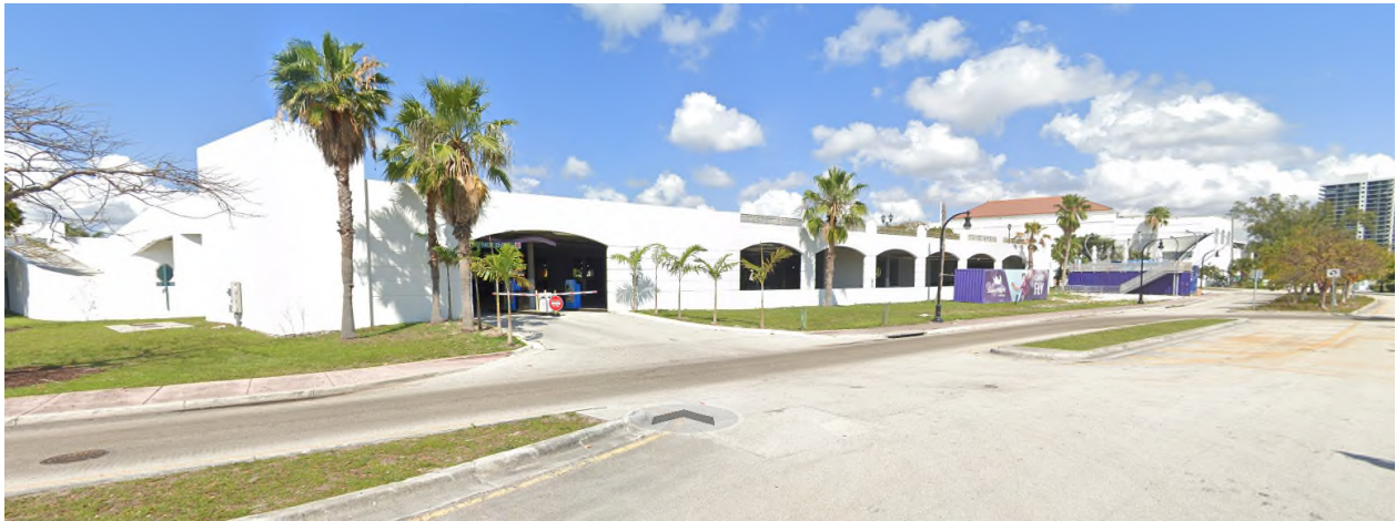
Looking west towards parking garage at southern exit
