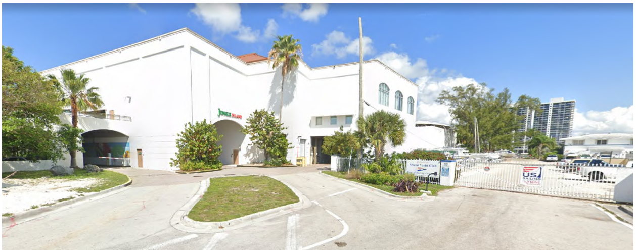
Looking west towards main building
