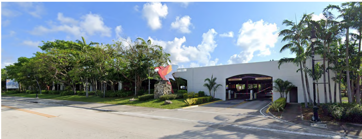
Looking east towards parking garage at southern entrance
