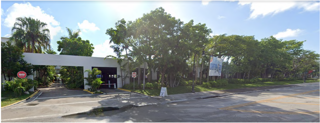
Looking east towards parking garage at northern entrance
