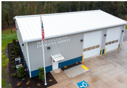
McCormick North EMS Substation
