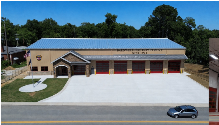
City of Barnwell Fire Station #1
