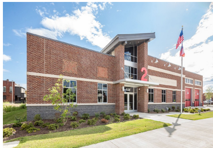
Augusta Fire Station #2
