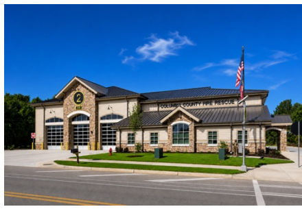
Columbia County Fire Station #2
