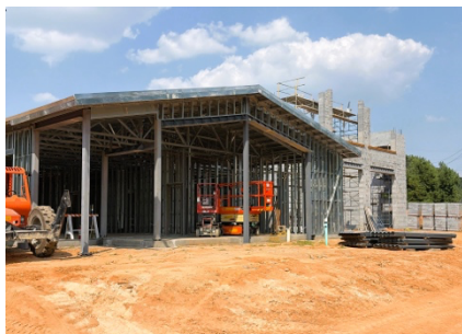
Augusta Fire Station #3
