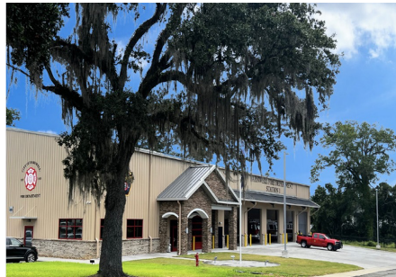
City of Barnwell New Fire Station
