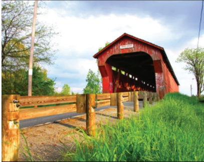
Swartz Bridge, Wyandot County, Ohio
