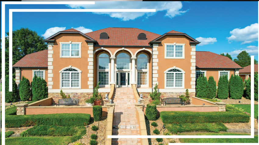
124 CROSS COMMUNITY ROAD BRISTOL, TN 37620 $3,495,000
