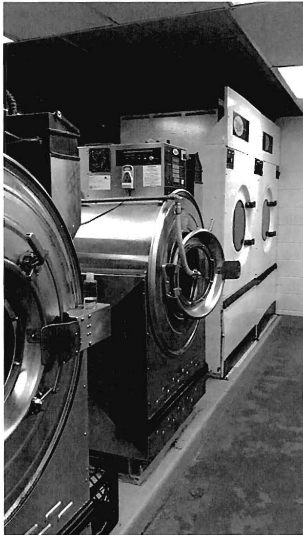
Figure 6: Photograph of the Laundry Room
