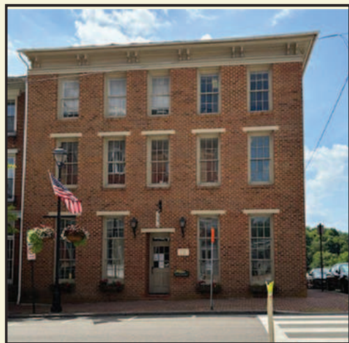
200 EAST MAIN STREET ABINGDON, VA Three story brick office building with two, two-piece restroom on each floor. Access to second and third floors is by stairway. Conference room and offices on each floor. The building is in good condition. $1,200,000
