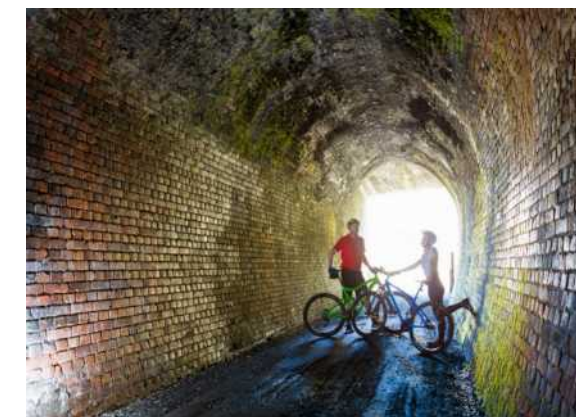
Example of Rail Trail Tunnel
