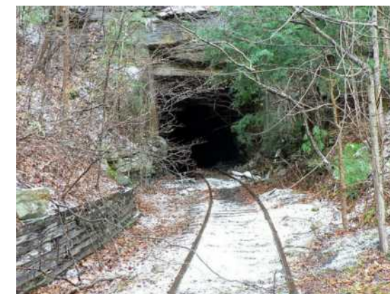
Abandoned Rail Tunnel
