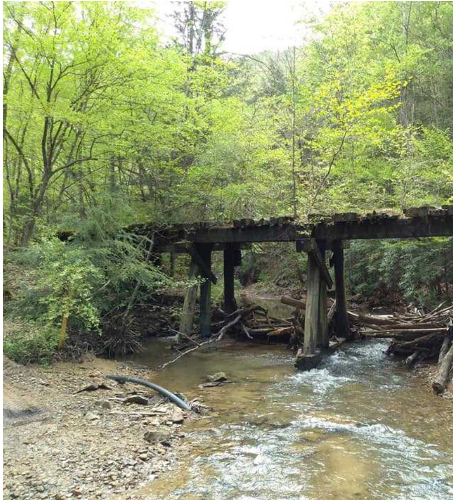
Existing Abandoned Bridge
