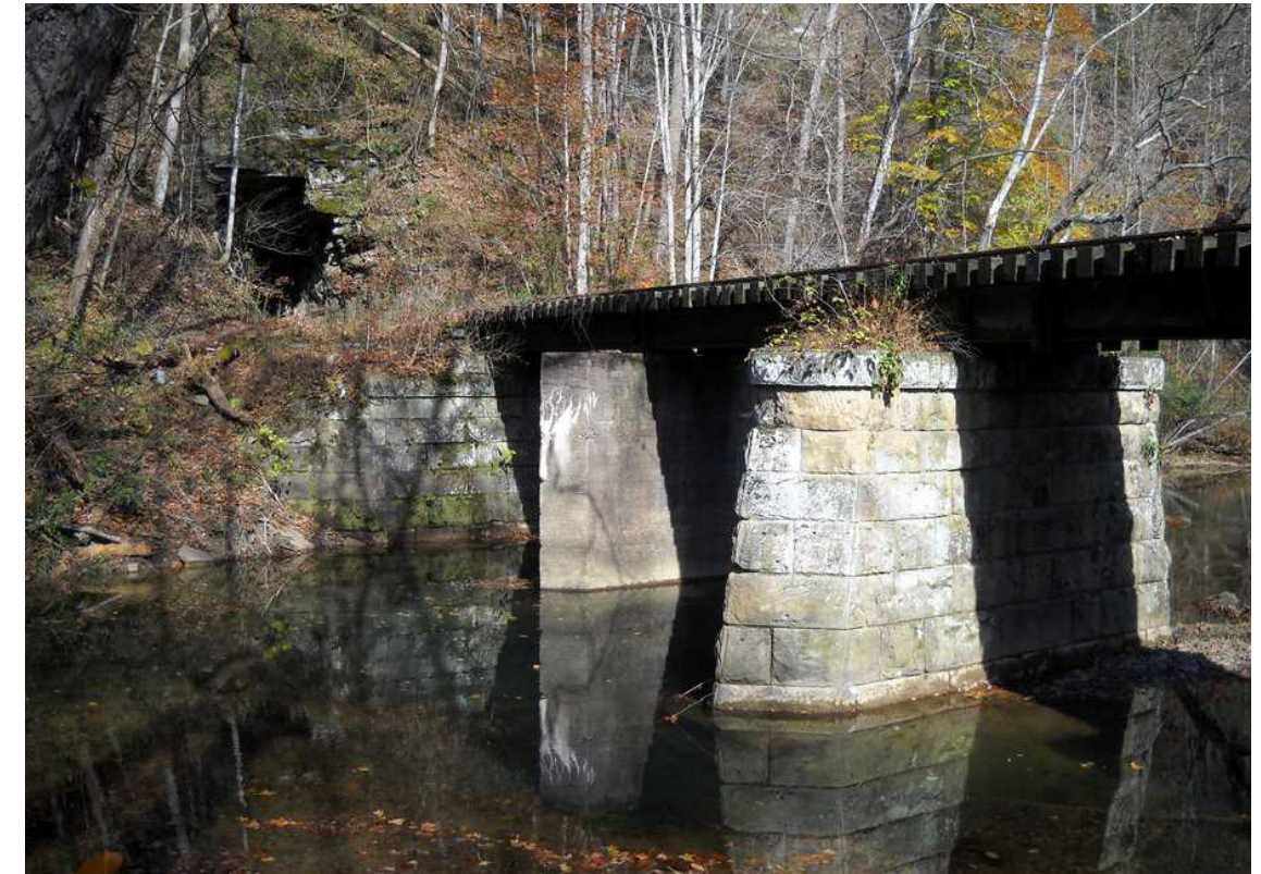
Existing Abandoned Bridge
