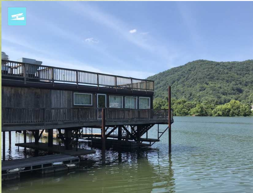
Chesapeake Marina and Boat Ramp Existing
