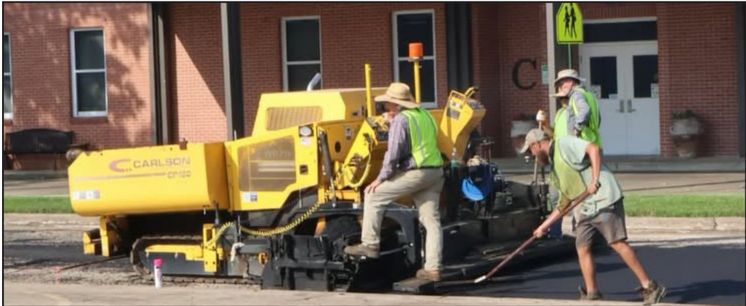
THE CITY of West Monroe’s Public Works crews are hard at work making road improvements across West Monroe as the city prepares for the upcoming school year. As work continues on streets throughout the city, West Monroe appreciates your patience around temporary lane closures and construction zones. Thank you to the city’s dedicated Public Works team for everything they do to keep West Monroe moving. (Courtesy photos)
