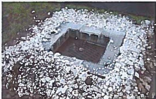
Figure 5.1. Excavated drop inlet protection with weep holes.
