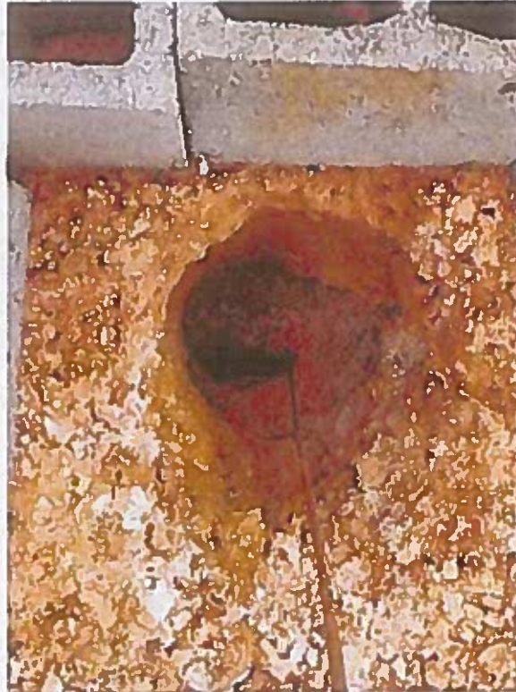
Photo 13. Damage offsite stormwater collection line
