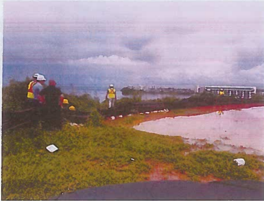
Photo 10. Intact silt fence and sandbag system with second silt fence installation on day of occurrence.
