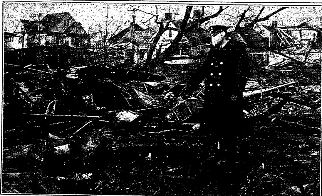
This picture was taken on McAdee street in the center of the area hardest hit by the tornado and gives a graphic idea of the extent of the damage done. It was at this spot that Mrs. J. B. Ayers and daughter perished.
