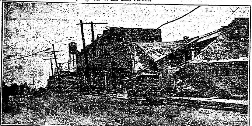
Scene on West Lee street, showing damages to Red Band Flour company and J. D. Wilkins, Inc., and also showing remains of Sinclair and National Oil companies in background.
