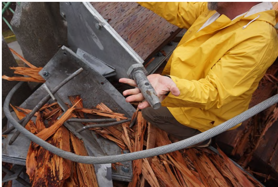
Photograph 27) – The connection at the apex.
