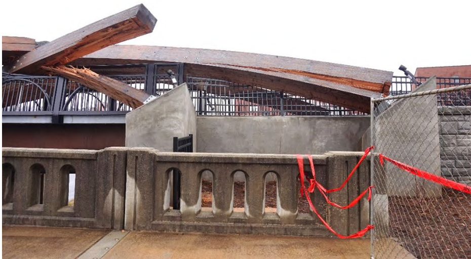
Photograph 2) – Northwest foundations for the arch base connections.
