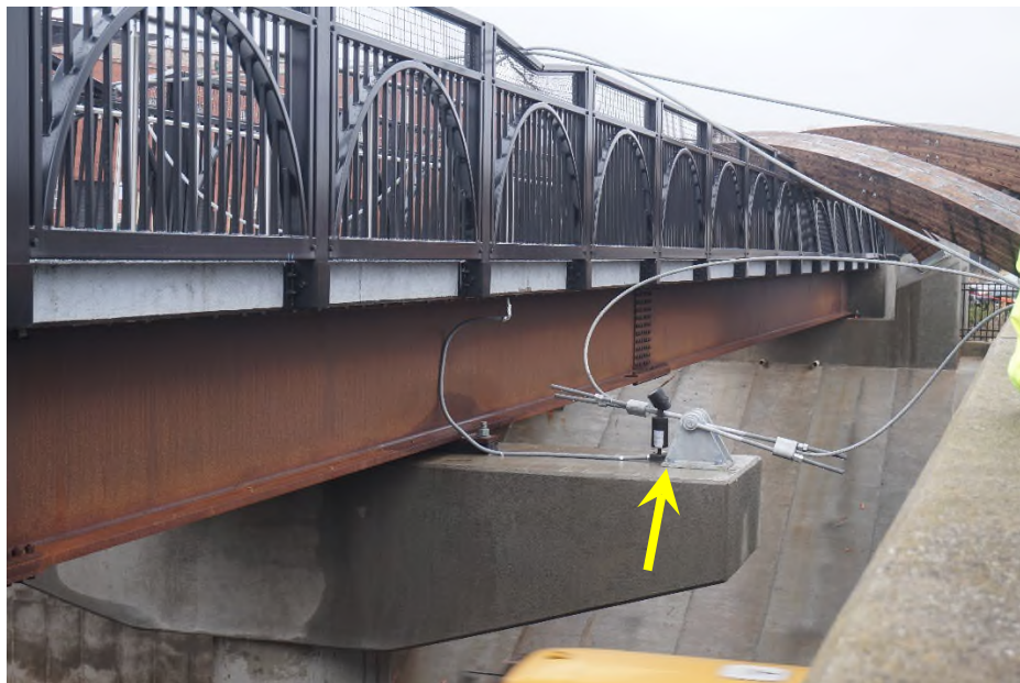
Photograph 22) – The anchorage of the two cables on the north face.
