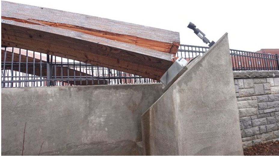
Photograph 3) – Closer view of the NW base connection of the upper arch.
