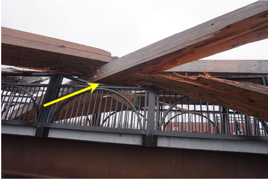
Photograph 25) – View of the lower arch.
