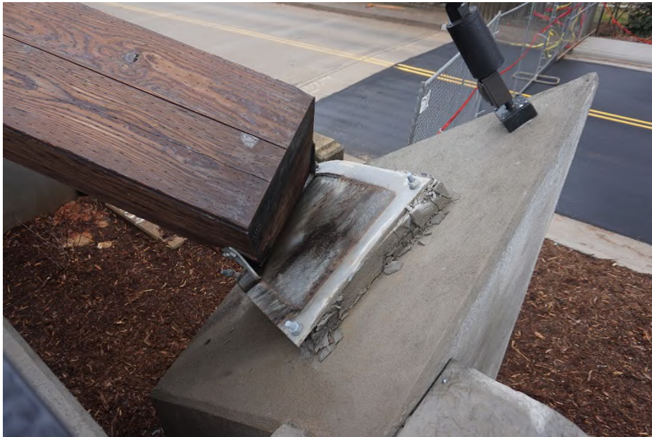
Photograph 10) – View of opposite face of Photo 8.
