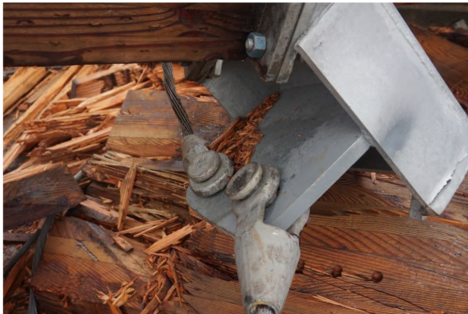
Photograph 17) – Another view of the intact cable bracket.
