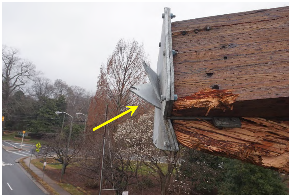
Photograph 28) – Part of the connection at the apex.
