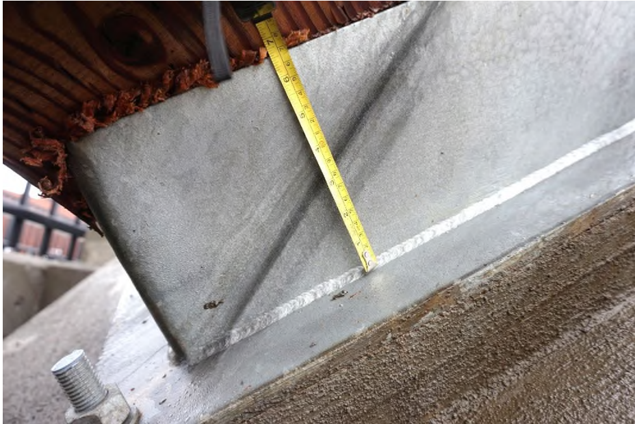
Photograph 6) – The steel base connection.
