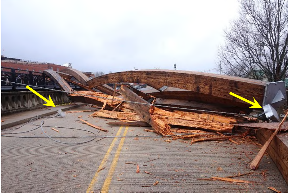
Photograph 13) – Cable connector on the left appears to be part of Steel Weld Assembly Mark S15. The one on the right is an intact steel cable bracket.
