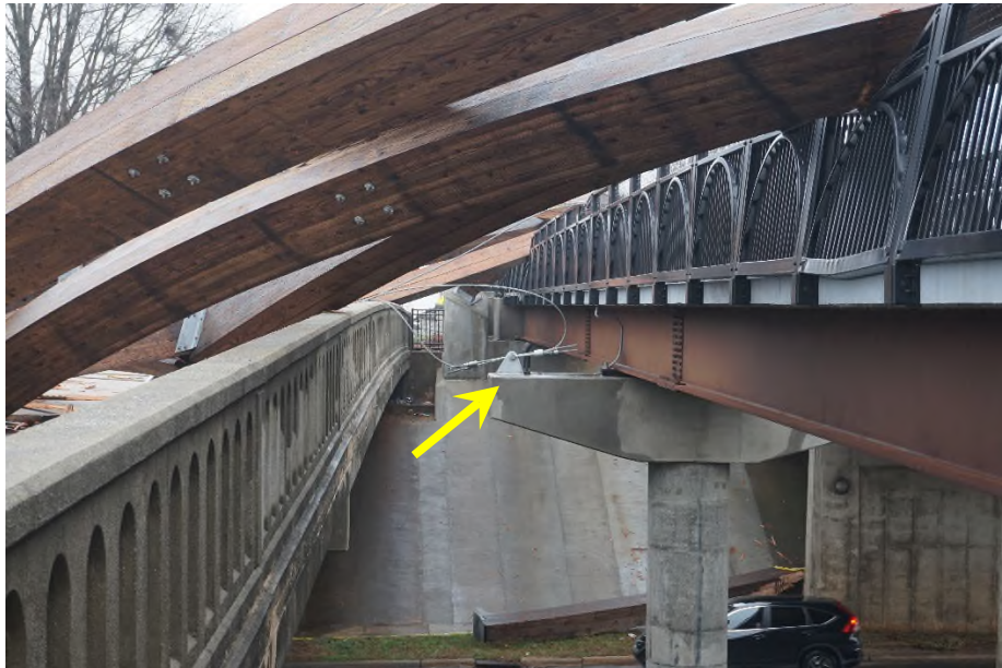
Photograph 12) – Example connection of the double guy wires on the north face.
