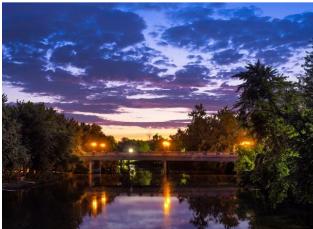
Harrison Street Bridge, from the St. Marys River
