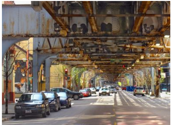
Conventional elevated transit
