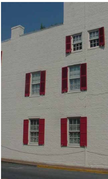
5-14 The first floor shutters on the house at 19 West 2nd Street are paneled, and the shutters on the upper stories are louvered. This practice allowed privacy from the street, but ventilation in the rooms above.
