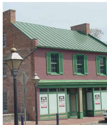
5-43 Only rarely does the entire roof structure require replacement. Most often, only the roof cladding—the outer skin of the roof—needs replacement. This standing seam metal roof at 46-48 South Market Street appears to have been replaced in recent years.
