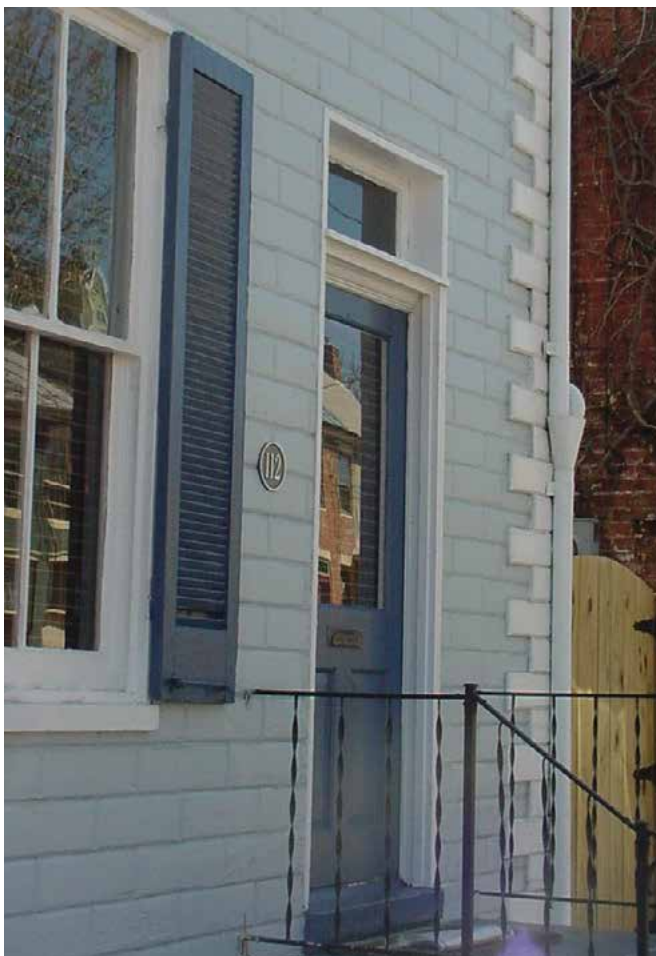
4-20 The house at 112 West 4th Street is sheathed in wood siding intended to resemble cut stone, with wood quoins at the corners. The wall treatment is a character-defining feature of this building.
