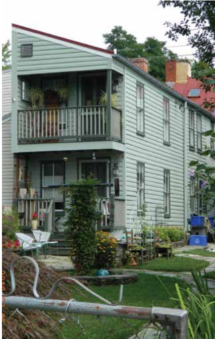
9-2 This two story addition on West 4th Street is subtly differentiated from the historic building with a vertical trim board.
