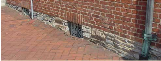
5-2 In many cases the material of the foundation differs from the primary wall material.
