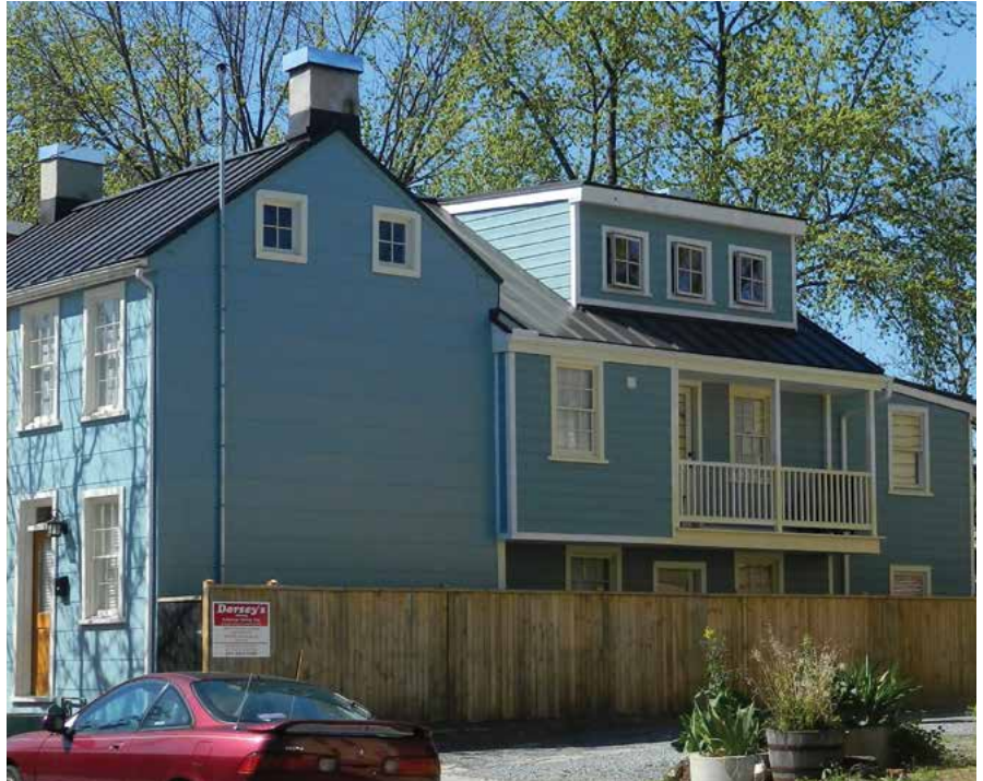
9-3 A shed dormer was added to the ell and a two story addition was constructed at the rear of this building on West 5th Street.
