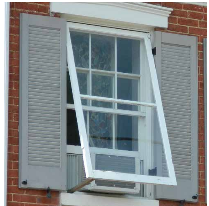
5-10 Historic wooden storm windows should be retained and preserved.
