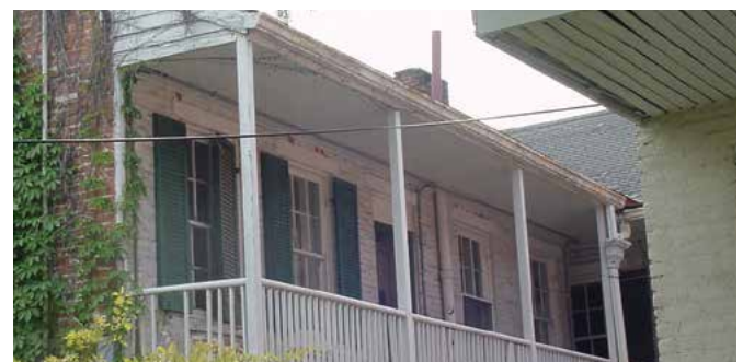
5-36 The porch ceiling on the right at 434 North Market Street shows the spacing of ceiling boards to allow ventilation. The porch ceiling on the left at 432 North Market Street is a solid board ceiling.
