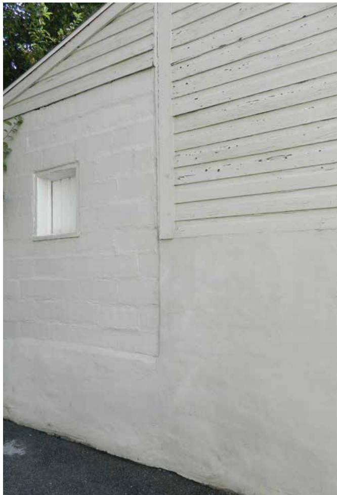
4-9 This foundation wall on Klineharts Alley has been parged and painted.
