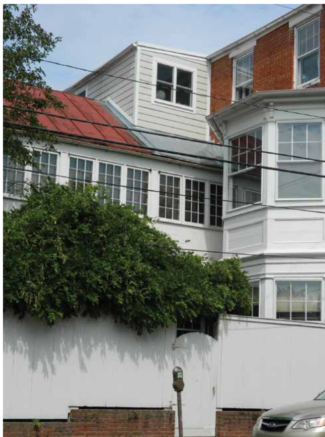
9-5 A modest frame extension at the third floor maintains the prominence of the historic structure's form.
