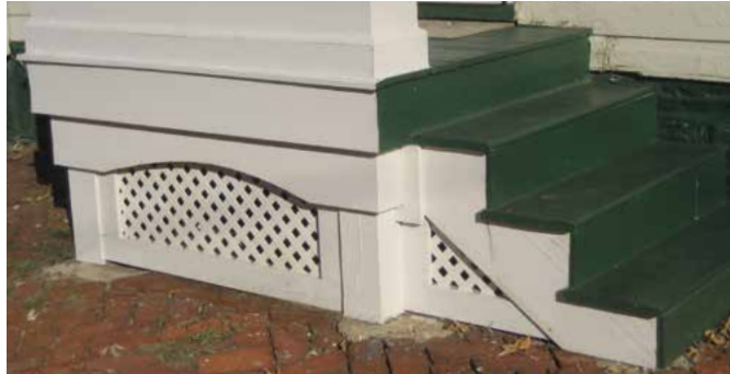
5-37 The underside of this porch at 39 East 4th Street shows the appropriate installation of lattice, with a wood frame at the periphery.
