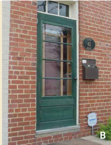
5-23 (A–C) These storm doors show some of the styles recommended by the Guidelines. These doors are modeled after the air-lock doors that are often seen as the outer door of a vestibule. The door on the left has a removable panel that allows the installation of a screen.
