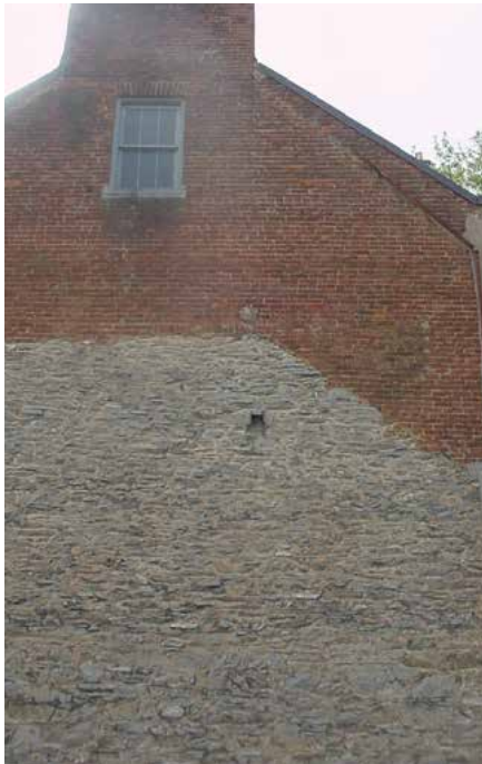
4-15 The stone portion of this wall is physical evidence that the building was initially a one-and-one-half story stone structure, later enlarged to two-and-one-half stories. Stucco was applied to the front of the building to unify the façade materials. The more modern brick on the newer construction is further evidence of the phased construction of this house.
