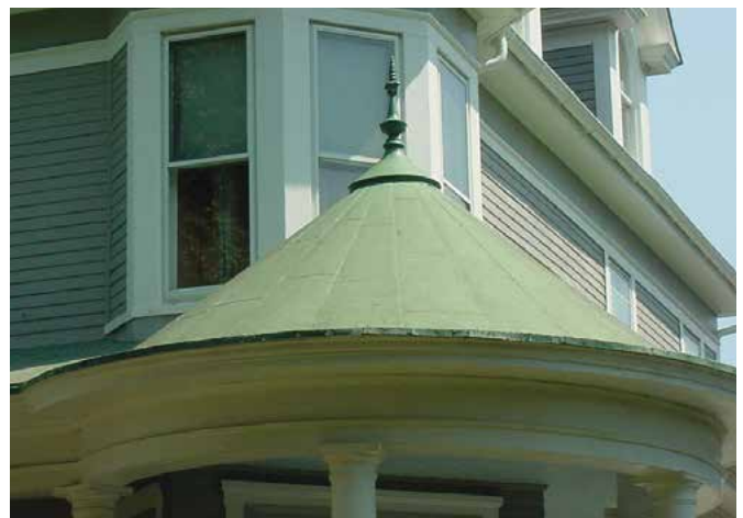
4-33 This flat-seam metal roof helps define the character of the tower on this house at 18 Clarke Place.
