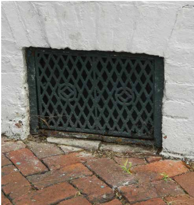
5-12 Historic metal grilles at a basement level window.
