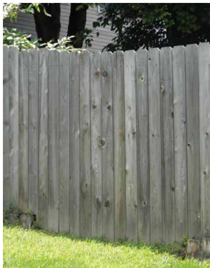
8-14 Solid board fence with "dog-ear" boards.
