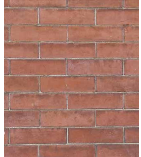
4-4 These tightly-spaced bricks with thin mortar joints are a twentieth century brick veneer.
