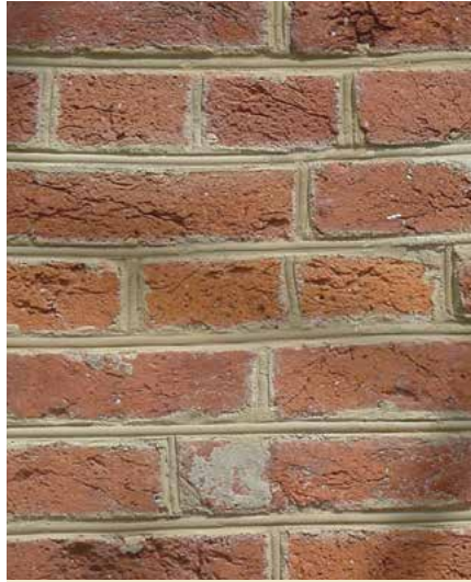
4-3 This wall laid in common bond has a beaded mortar joint.
