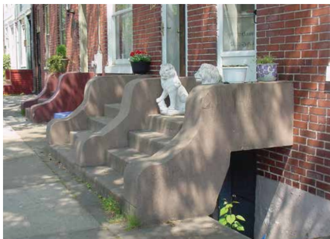
5-31 The concrete stoops at 113-117 West 4th Street are notable for their curved cheek walls.
