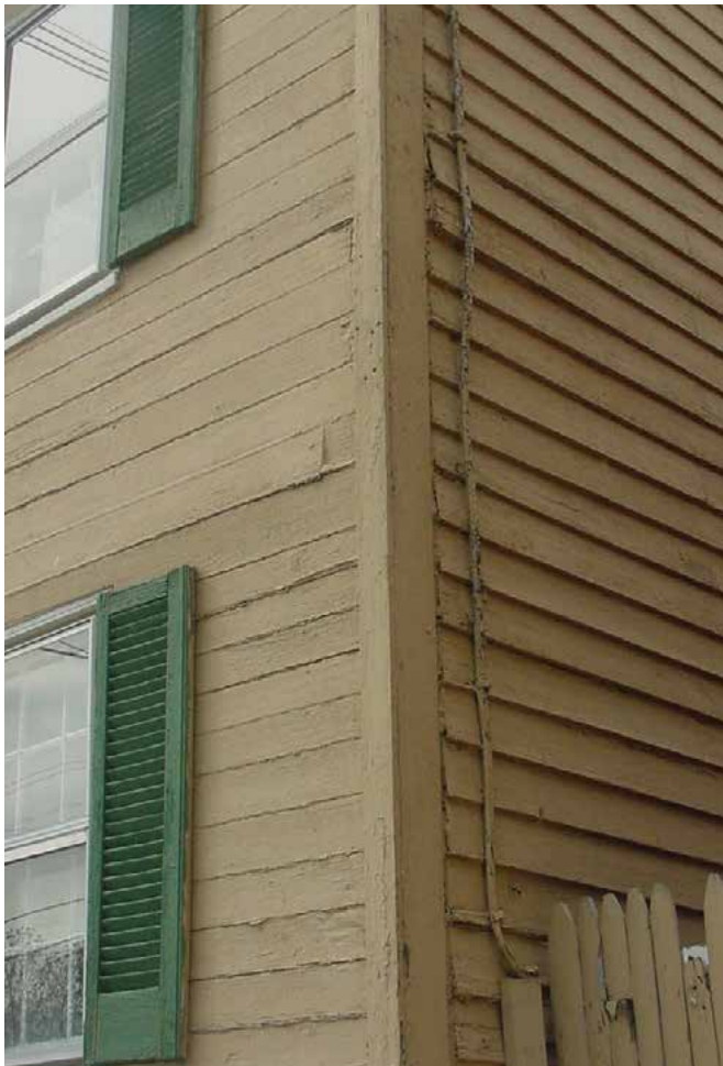
4-18 This house at 101 East 6th Street exhibits two kinds of wood siding used on historic Frederick buildings. The side wall is sheathed in simple lap siding, sometimes known as clapboards or bevel siding. Tongue-and-groove wood siding is evident on the front of the house.
