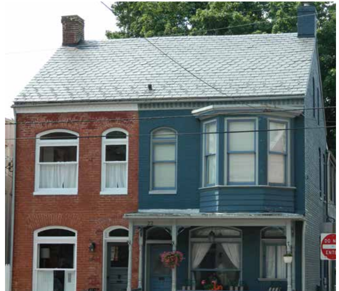
4-31 This slate roof on West 4th Street exhibits slate of various shapes.
