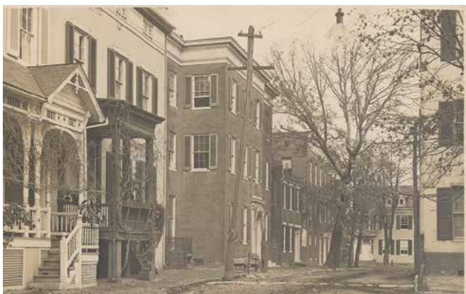
4-22 Historically, lattice was either square or diagonal-cut and was installed with a frame. The Commission requires lattice to be framed, as shown on this c.1905 photograph of 111 Record Street. Courtesy of Stanley Sundergill.
