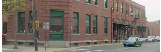
5-3 The alteration of openings can visually disrupt a façade, including the adaptation of a door to a window, as seen at the corner of 200 East Patrick Street.
