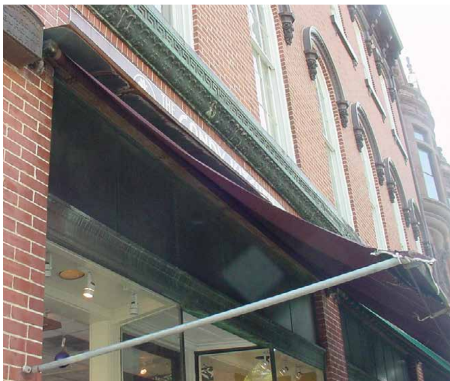
5-52 The awnings at 52 North Market Street resemble those in historic photographs. Although the fabric recently was replaced, the traditional hardware still is in use.
