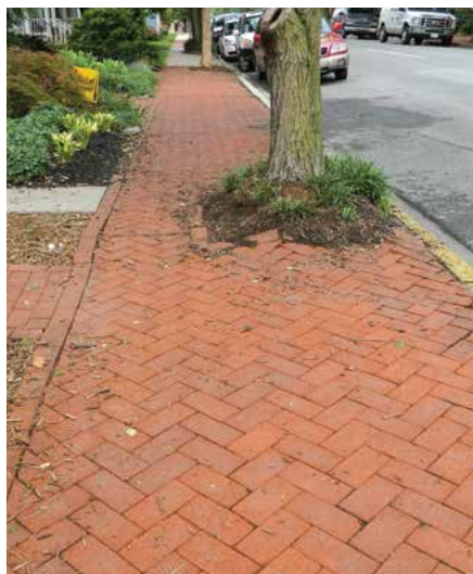
8-22 Herringbone paving on East 3rd Street.
