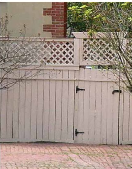
8-13 Solid board fence with lattice top.
