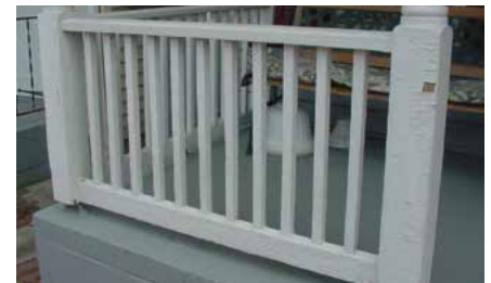
5-33 The parts of a balustrade are shown on the porch at 216 East 6th Street. Balustrades and porch floors may deteriorate sooner than other porch components. Replacements must be in keeping with the existing porch.
