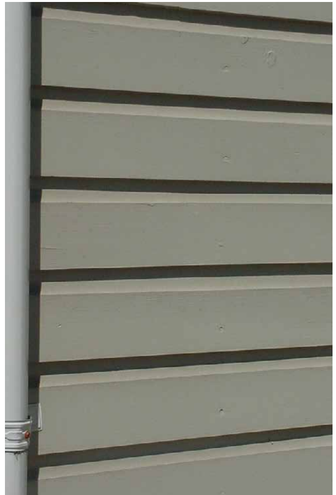
4-19 The most common wood siding in the Historic District is known as German lap siding . Typically the concave upper edge of the board fits into a groove in the board above. In some places this siding is known as drop , Dutch lap , cove lap , or novelty siding .
