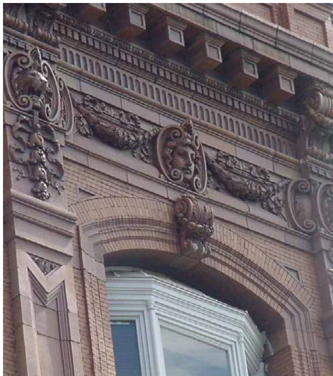
4-30 This terra-cotta detailing contributes to the significance of the building at 2 North Market Street.
