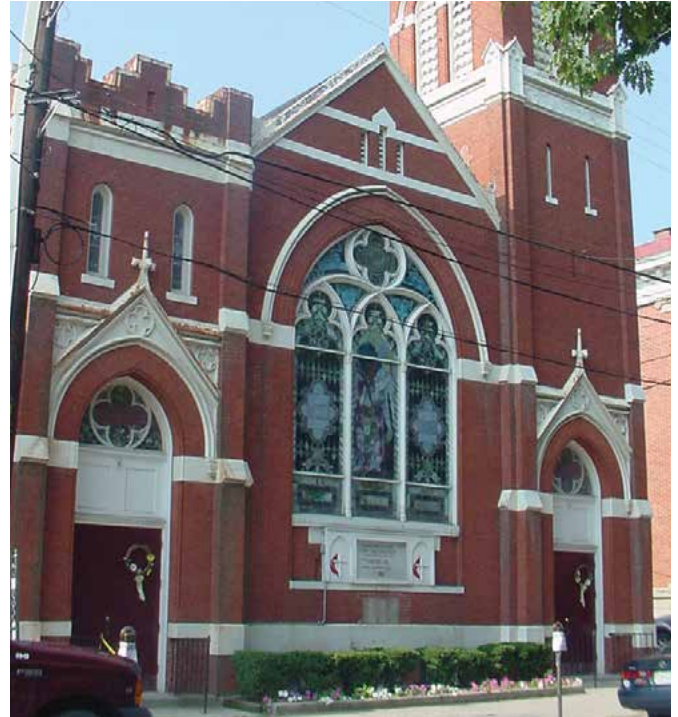
4-27 The stained glass windows at Centennial Memorial United Methodist Church at 8 West 2nd Street are character-defining features that require special maintenance. The lead between the panes of stained glass, known as cames, needs to be kept in good condition to hold the glass in place and prevent water penetration.
