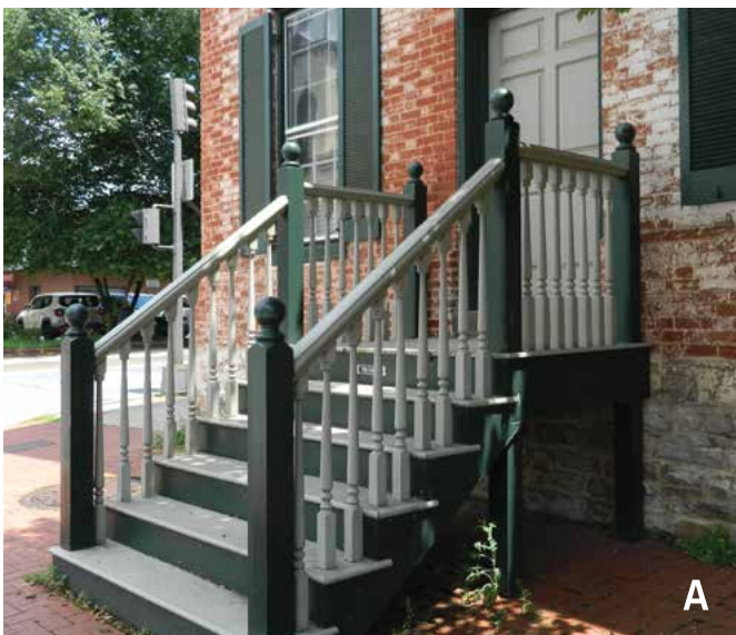
5-29 (A–B) Stoops are entry features that are smaller than porches. Whether plain or elaborate, a door stoop should be in keeping with the remainder of the building in materials, style, and embellishment.
