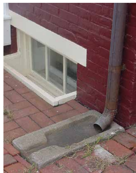
5-51 The splash block at 152 West Patrick Street is a character-defining aspect of the drainage system on the house.
