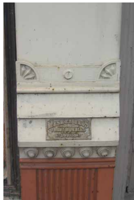
4-25 The metal storefront at 36 South Market was manufactured by the Mesker Brothers of St. Louis. This character-defining metal feature requires painting on a regular basis to deter rust.
