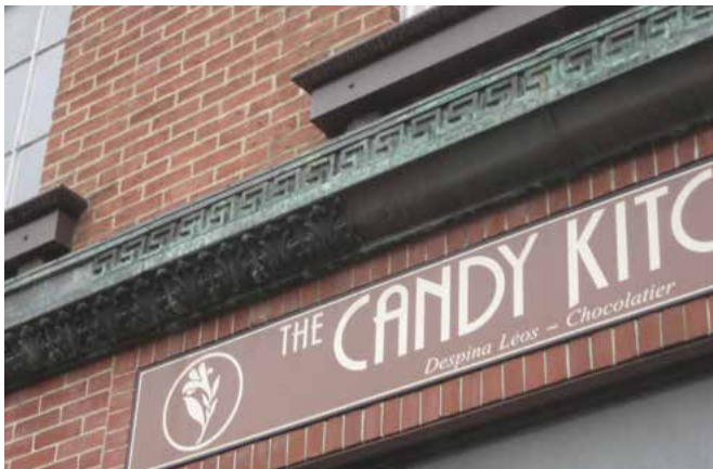
4-23 The metal fret pattern, although slightly deteriorated, adds richness to the building at 52 North Market Street.
