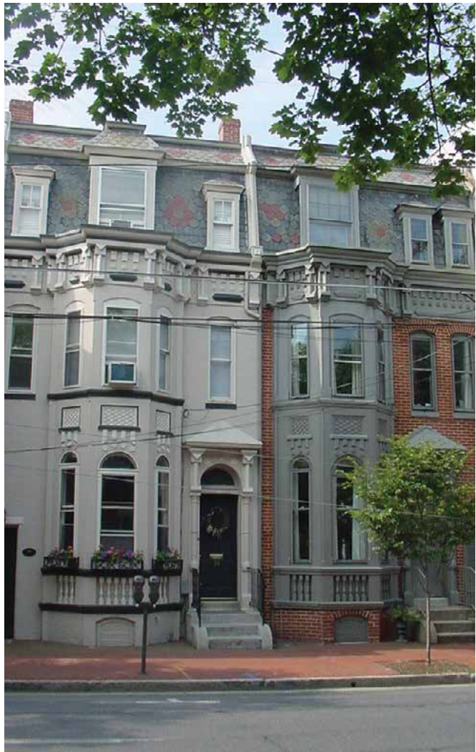
4-14 Paint on unpainted masonry is regulated by the Historic Preservation Commission. The unpainted unit on the right, 32 East 3rd Street, cannot be painted without Commission approval. The unit on the left, 34 East 3rd Street, which already is painted, can be repainted without Commission approval.
