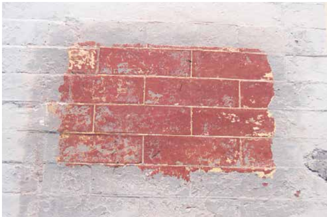
4-11 Before the Commission approved the removal of the paint at 118 West 3rd Street, it required a test patch. The Commission determined that the twentieth century brick and mortar would not be harmed by the removal of the paint using the tested product.
