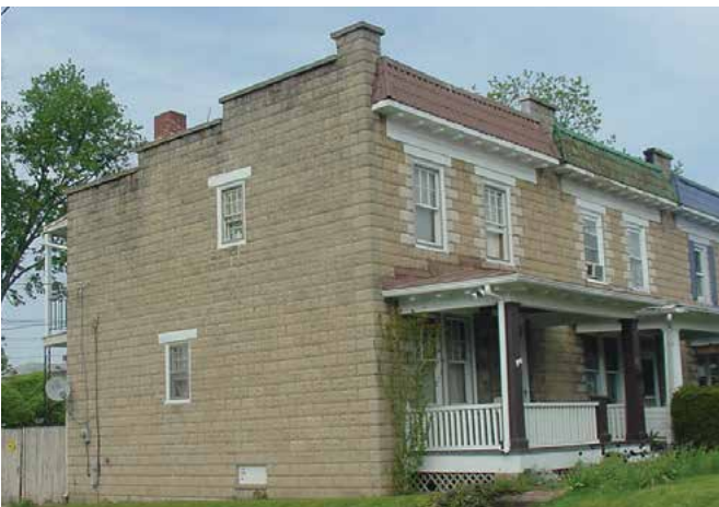
4-13 The twentieth century row houses on East 7th Street were faced with split-face block. Few buildings in the Historic District have terra-cotta roofing, as seen on these pent roofs.
