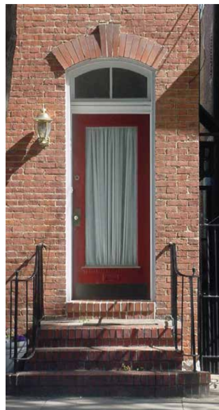
5-16 The essential components of an entrance are evident at the main entrance to 123 West 2nd Street.
