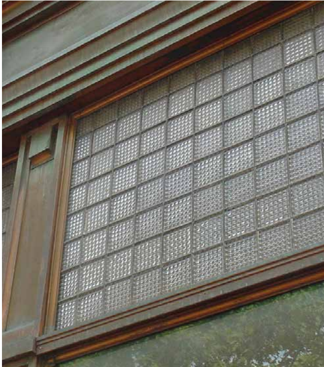
4-26 Glass needs to be replaced when broken and structural elements need to be painted, caulked, and repaired on a regular basis. The building at 48 East Patrick Street features a prismatic glass transom.
