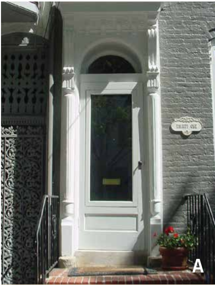
5-23 (A–C) These storm doors show some of the styles recommended by the Guidelines. These doors are modeled after the air-lock doors that are often seen as the outer door of a vestibule. The door on the left has a removable panel that allows the installation of a screen.
