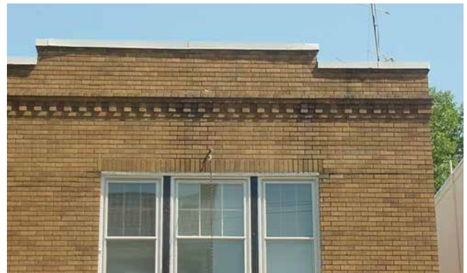
5-4 The stepped parapet at 107 East Patrick Street has corbelled brick detailing at the cornice line. Parapets often are used to conceal mechanical equipment on additions and infill construction.
