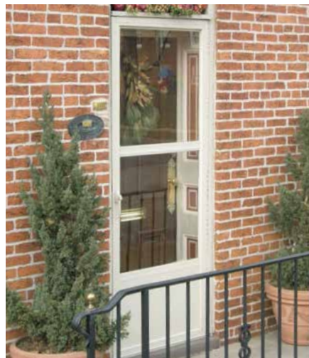
5-24 This metal storm door originally had an aluminum finish, but its rehabilitation included painting, which eliminated the metallic finish the Guidelines do not sanction.
