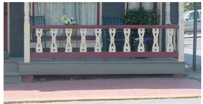
5-35 This house has cut wood balusters and turned porch posts.
