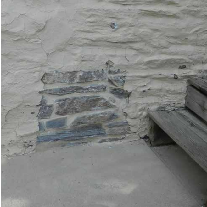
4-10 The removal of stucco and parging require approval from the Historic Preservation Commission and must not damage the underlying material. A test panel is typically required.
