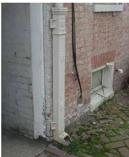
5-50 Although often considered ephemeral building elements that need periodic replacement, some downspouts are built for longevity, such as this cast iron downspout boot at 148 West Patrick Street.
