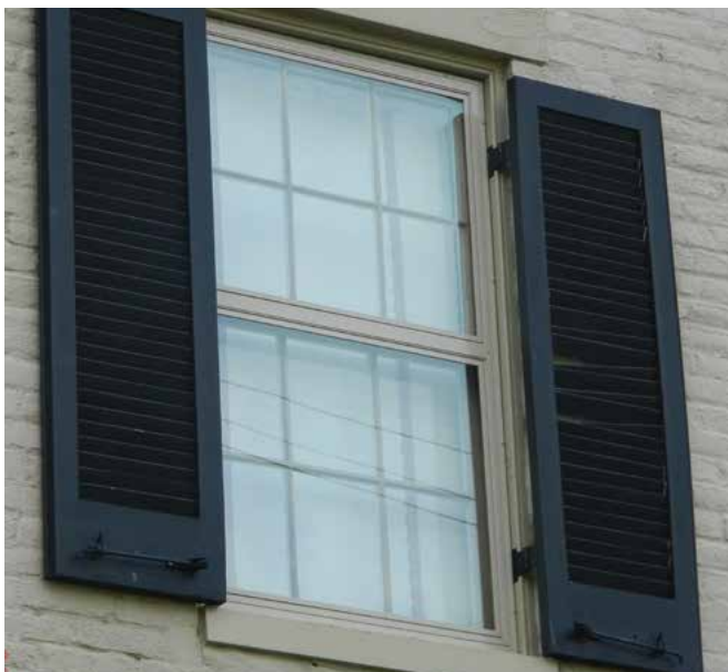
5-9 The narrow frames of this storm window are unobtrusive, and the mid-rail of the storm window is aligned with the meeting rail of the window. Storm windows add energy efficiency and may protect the wood and glass of historic windows.
