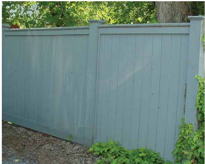
8-12 Solid board fence with cap board.
