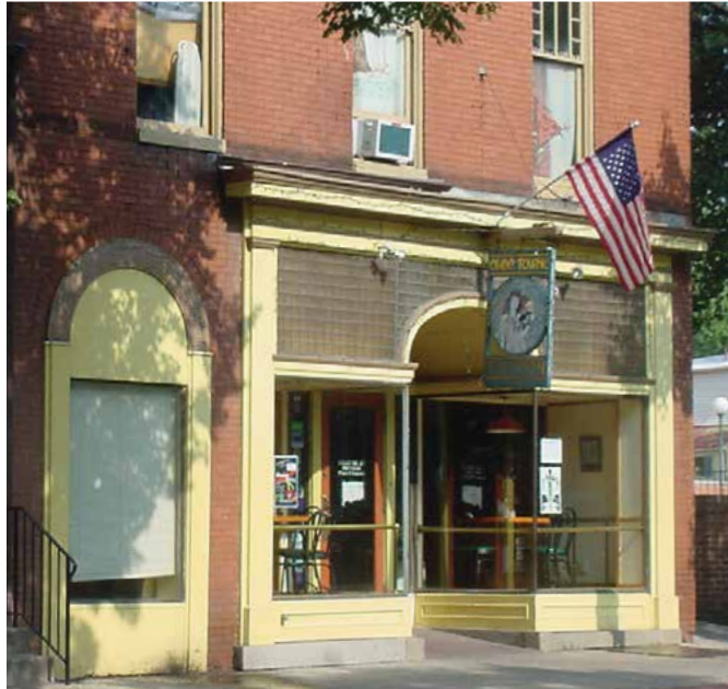
6-2 This storefront at 325 North Market Street illustrates the typical features of retail commercial buildings, including a centered and recessed door, display windows, and wide transom.
