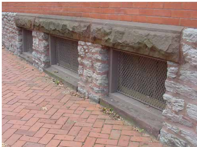
4-1 Stone architectural details, such as the lintel on this building owned by the Evangelical Lutheran Church at 35 East Church Street, is a character-defining masonry feature.
