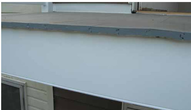
4-21 The edge of the back porch floor at 246 East 6th Street reveals the tongue-and-groove flooring that was typical of wood porches.
