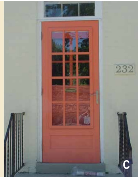
5-23 (A–C) These storm doors show some of the styles recommended by the Guidelines. These doors are modeled after the air-lock doors that are often seen as the outer door of a vestibule. The door on the left has a removable panel that allows the installation of a screen.
