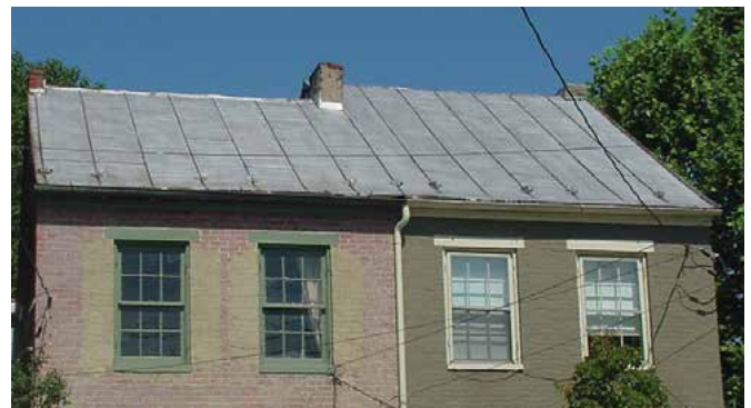
4-32 Traditional standing seam metal roofs, like this one at 101-103 North Bentz Street, have been a popular roofing material in Frederick for many years. The snow birds or snow guards at the bottom edge keep snow from sliding off the roof.
