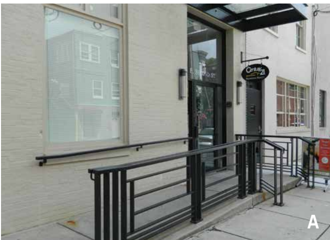
7-4 (A–B) Ramps are one way to provide an accessible entrance to building.
