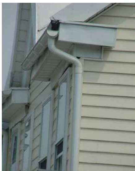
5-49 Half-round gutters and round downspouts, shown at 200 East 6th Street, are generally appropriate in the Historic District.
