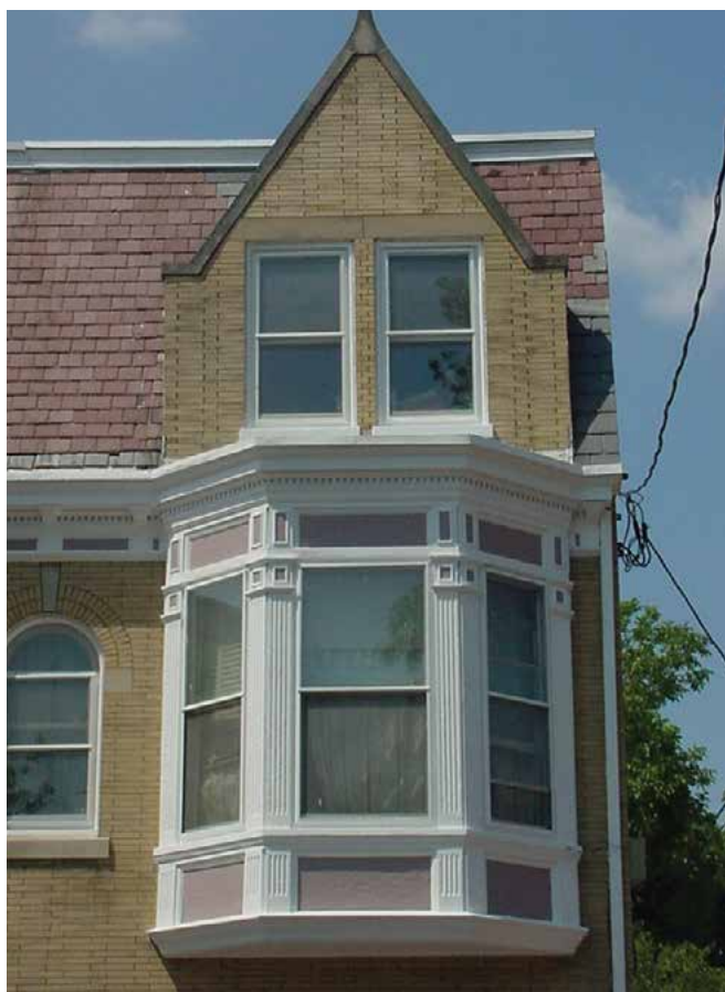
5-44 The wall dormer that rises above the oriel window at 15 East 2nd Street is a character-defining feature, as are all historic dormers.
