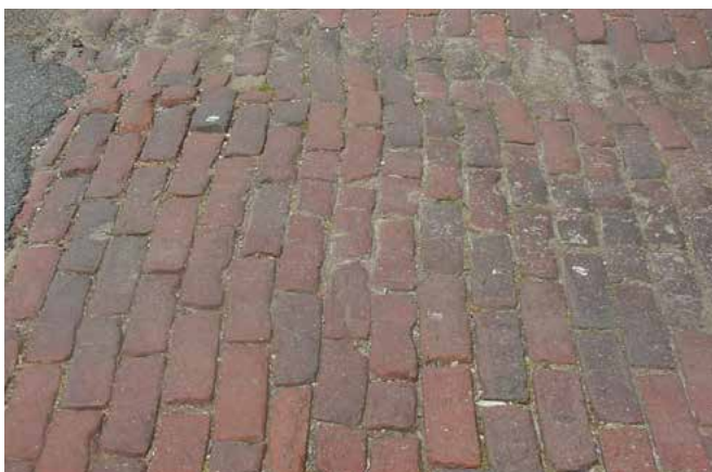
4-35 This brick near All Saints Street is laid in a running bond pattern.
