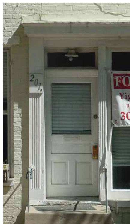
5-19 Doors with half-lights (a fixed pane of glass in the top half) are most common as back doors. The door at 201 East 3rd Street has three panels, a fairly unusual door style for the front elevation.
