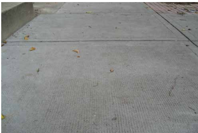
4-36 The sidewalk in front of 121 West Second Street exhibits the dimpled finish, a common treatment in earlier periods.
