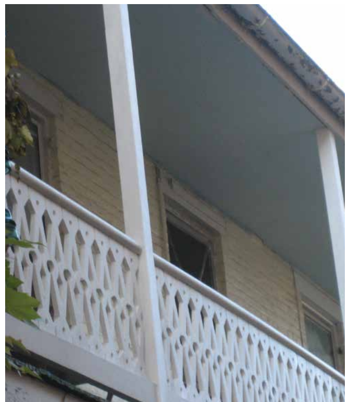
4-29 This porch ceiling at 121 West 2nd Street is plaster, a treatment generally reserved for porches on upper levels.
