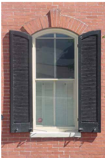
5-15 The shutters on the house at 11 East 2nd Street are curved at the top to correspond with the window opening. If these shutters need to be replaced, the new shutters will have to fit the opening and have the same details, dimensions, and hardware. Sometimes old shutter hardware can be re-used.
