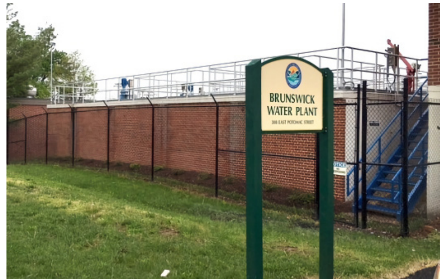
Located at 300 East Potomac Street just southwest of Downtown Brunswick, the Brunswick Water Treatment Plant withdraws and processes water from the Potomac River.
