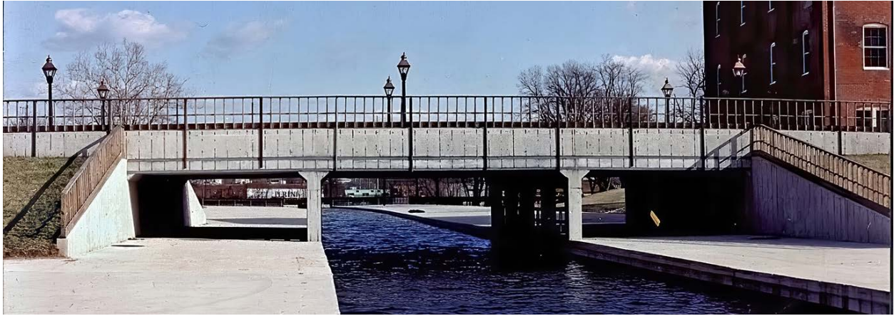
The Carroll Street Bridge in 1993.
