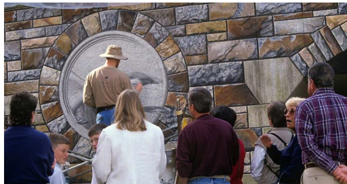
The final major feature of Community Bridge underway in 1997.
