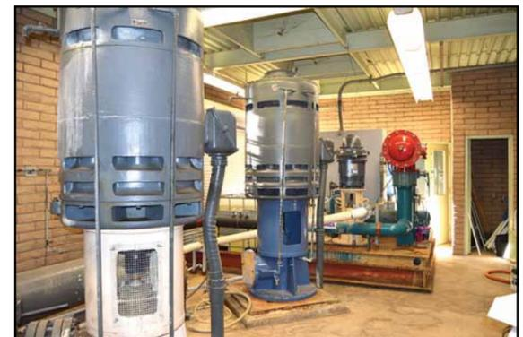
The pumps for the fountain were evaluated as part of the study by Black and Veatch. Check valves on the pumps are currently being replaced.
