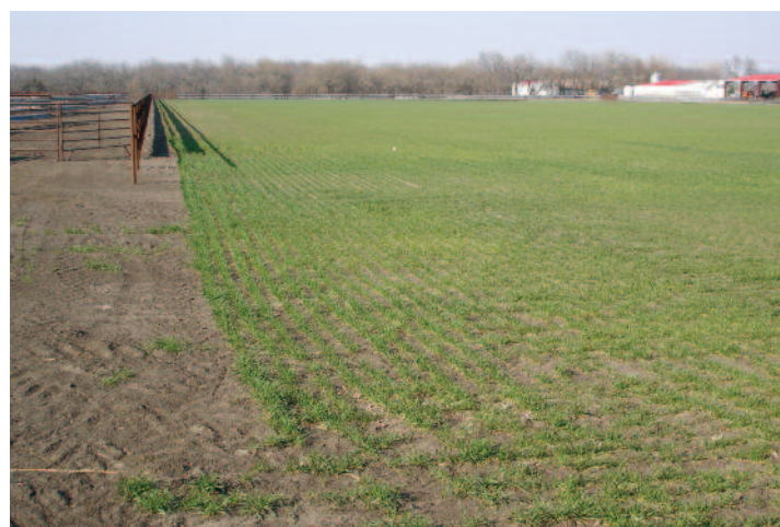
Settling bench and vegetated treatment area below a drovers alley.
