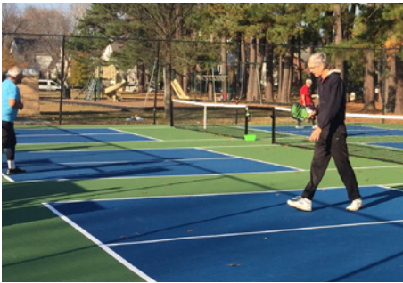
At Memorial Recreation Park in Fredericksburg, VA, new pickleball facilities were built to help meet the growing demand.
