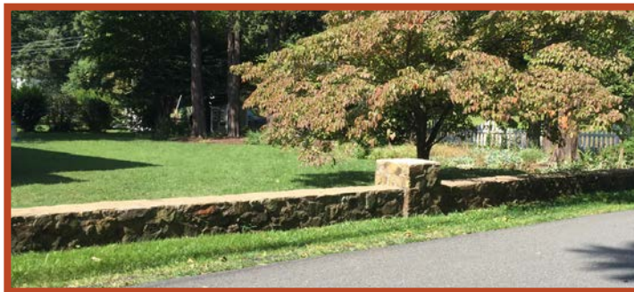
STONE COLUMN & WALL
