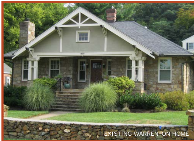
Exposed Rafter Tails and Knee Braces
