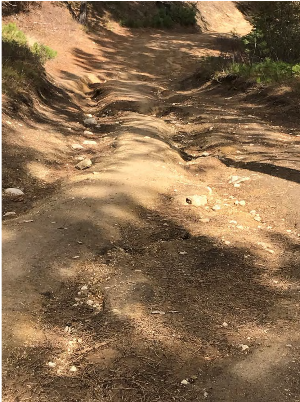
3-22-2024 view of FR 74964, the access road to trail 511 and the Westside project road to unit 2c. No maintenance has been done since the Westside commercial harvest concluded, and it is now impassible to passenger cars.
