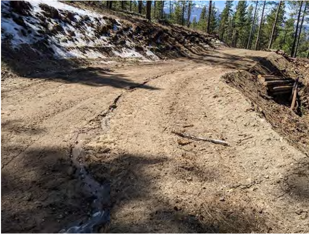
Road failure with logs piled in break in roadway from two angles.
