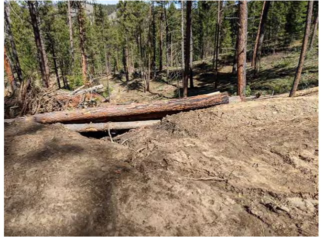
Road failure with logs piled in break in roadway from two angles.
