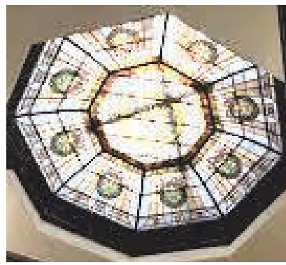
City Hall Skylight
