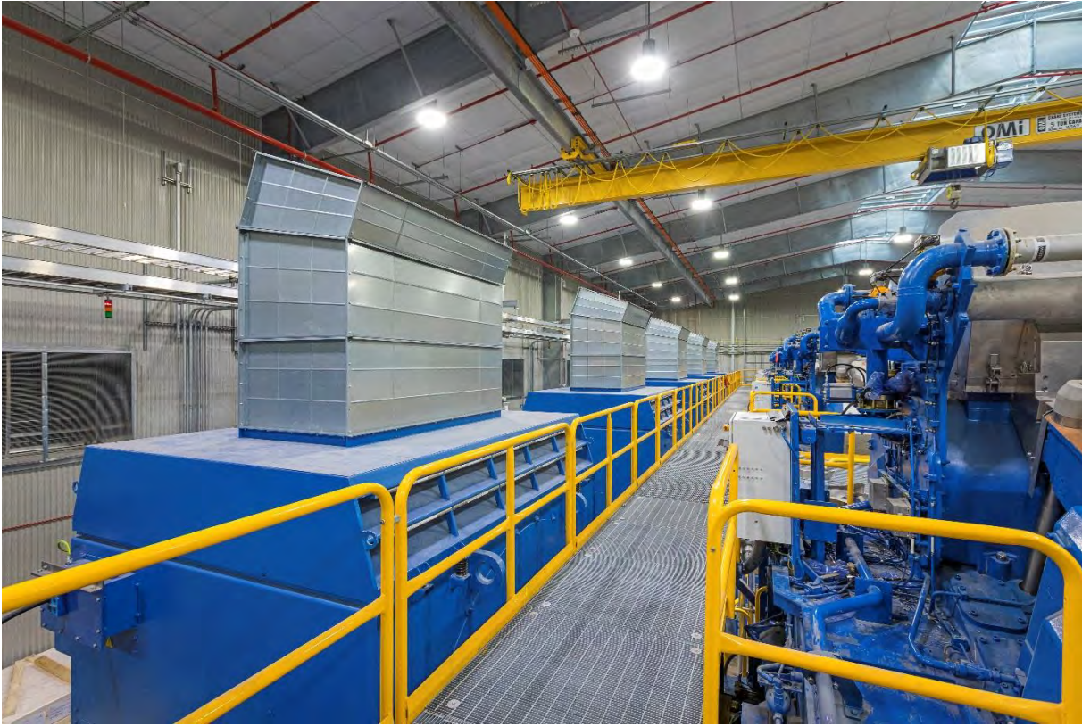
DEC North Hall Generators
