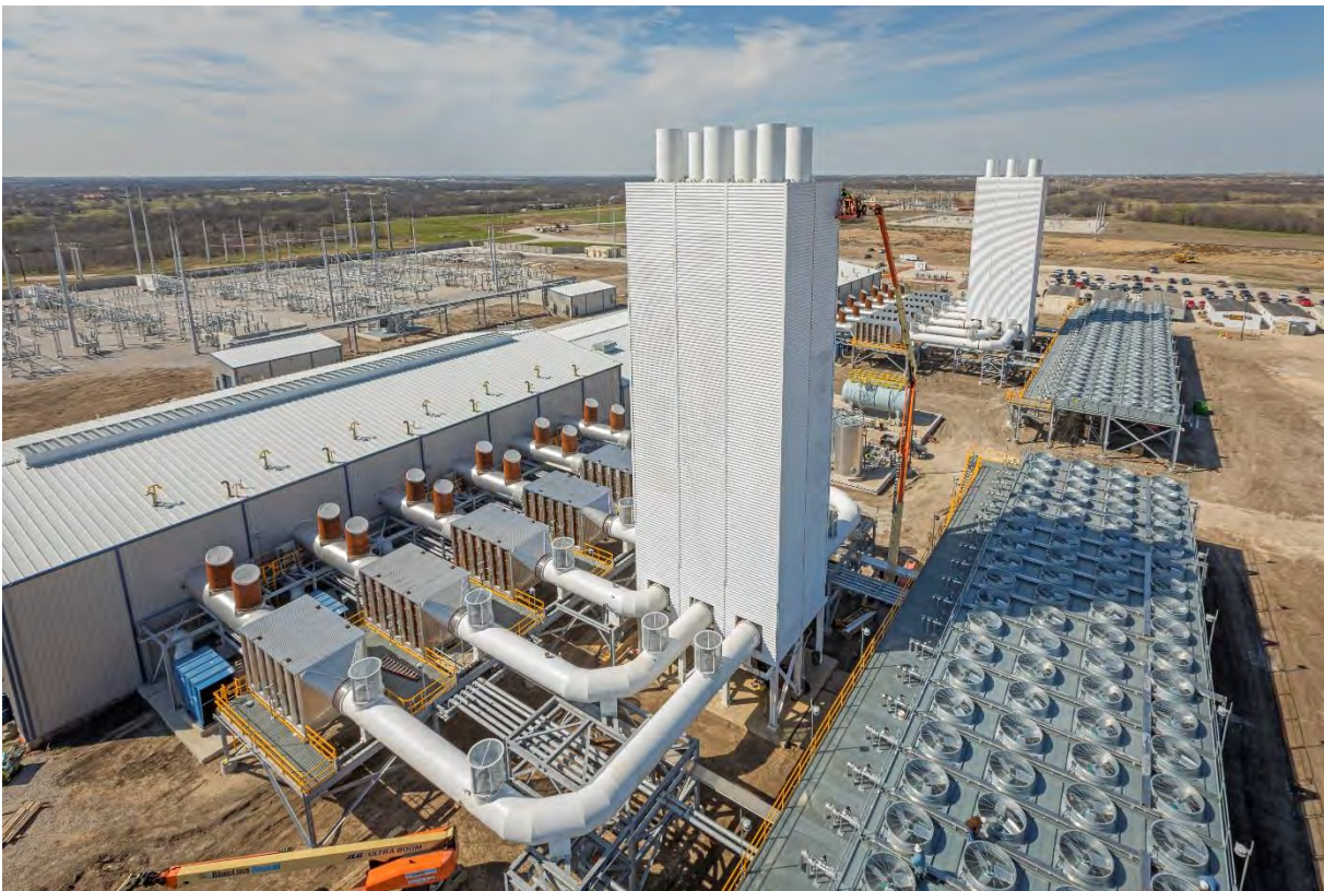
Aerial View looking Northwest
