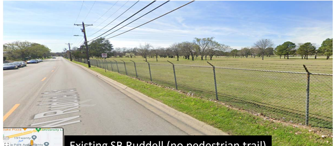
Existing SB Ruddell (no pedestrian trail)
