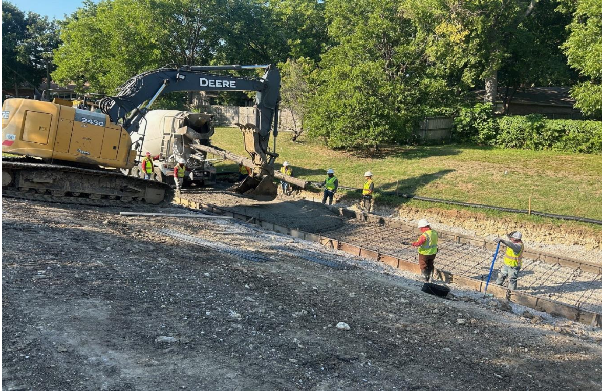
City of Denton Excavator
