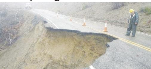
During this past winter and spring heavy rains, Gardner Ridge Road near Brookings collapsed, leaving only one lane available for travel. Photo courtesy **Oregon Emergency Management.**
