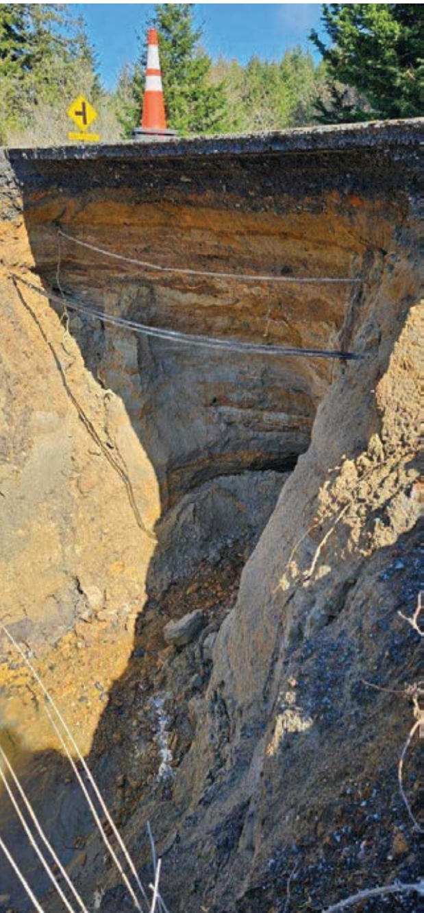
Erosion: The culvert under U.S. Highway 101 at Bearhead Mountain Lane is located about six miles south of Bandon. The two-foot-diameter pipe is about 20 feet below the road surface.
