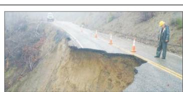
Gardner Ridge Road is the only access for 10 families. During the heavy spring rains, the roadway collapsed, leaving only one lane available for travel. Photo courtesy of OEM
