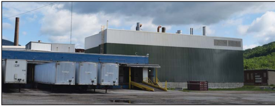
The new owners of the White Mountain Paper Co. in Gorham plan to demolish 40 percent of all its buildings' exteriors and remove 25 percent of what's inside, cutting overhead costs so its paper (tissue) machine (inside boxy building, right) turns a profit. (EDITH TUCKER PHOTO)
