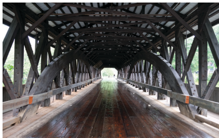
The arch and trusses can be seen inside the Saco River Covered Bridge in Conway.
