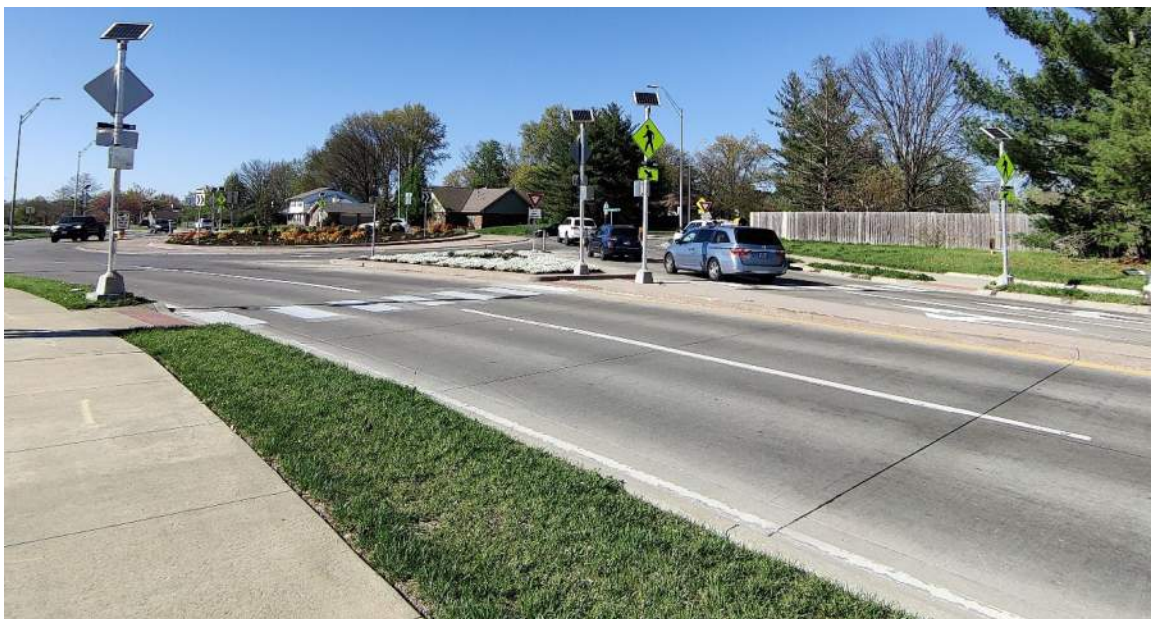
Photograph 7: Forum Blvd & Green Meadows (RRFB at Roundabout)
