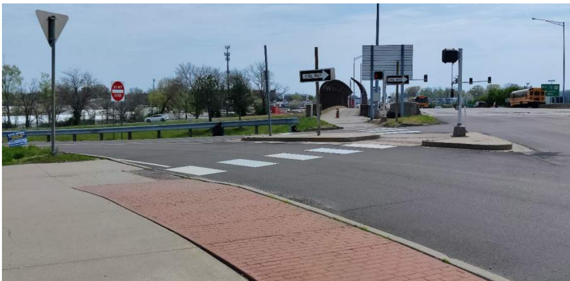
Photograph 15: Providence Pedestrian Bridge
