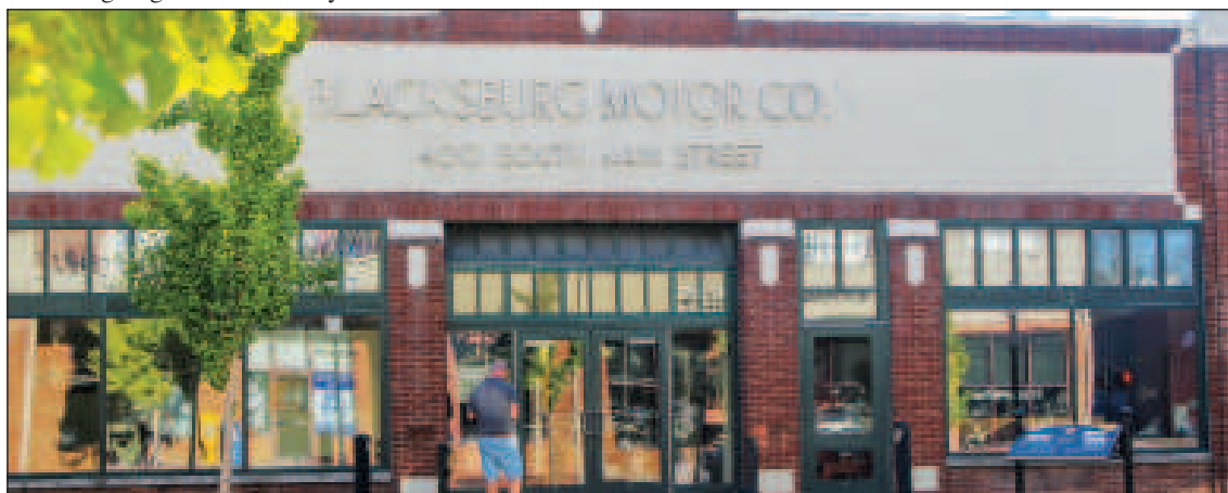
The Blacksburg Motor Company Building sits on Main Street in the afternoon light, with citizens of Blacksburg walking up and down the street to visit the building, Oct. 18, 2016.
