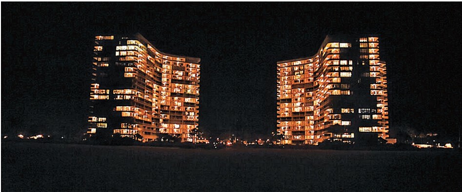
South Seas West Towers One and Two BEFORE the Lighting Retrofit Grant.
