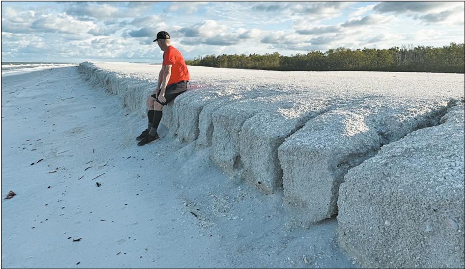
Photos by Maria Lamb Taken on August 24, 2025, a view of a series of water rivulets causing erosion on the berm, which was completed in April 2025.
