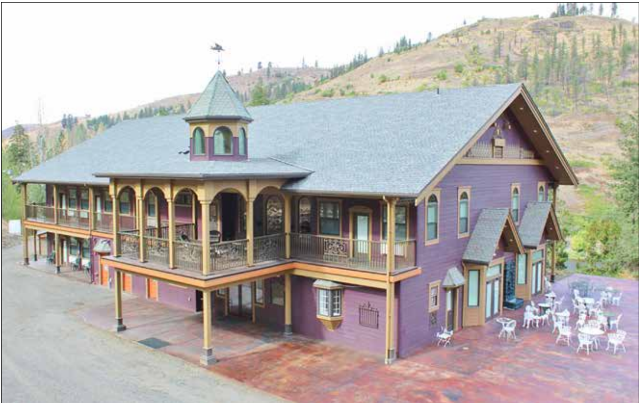
The front entrance of the nearly completed Hearthstone Lodge
