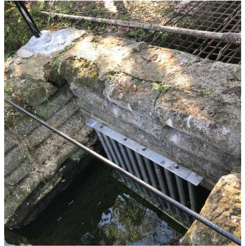
View From Hippo Enclosure Side Weir panel installation in December 2017
