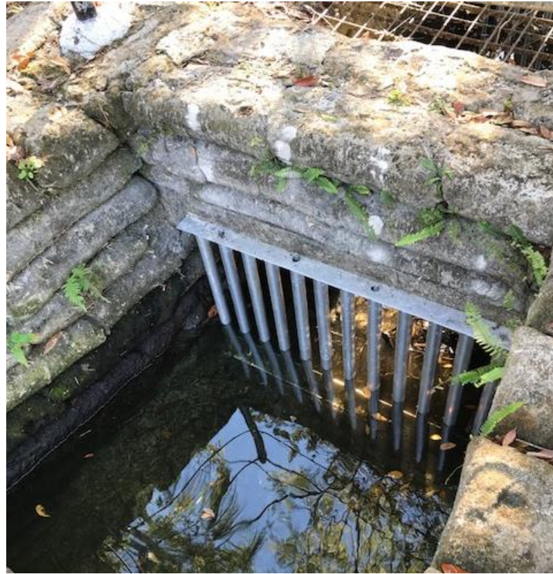
View From Hippo Enclosure Side Weir panel installation in December 2017
