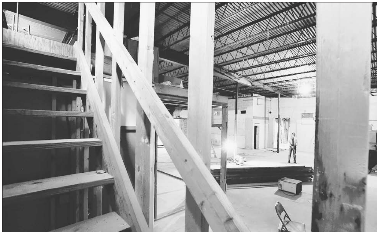
Citrus County Facilities Management Director Carl Hall stands in the space Monday, Oct. 25, discussing plans for the project.
