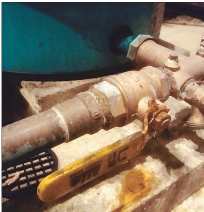
This is my main water shutoff valve. Do you know where yours is? Do you know if it works? Do you know how to de-pressurize your water lines? You probably don't.
