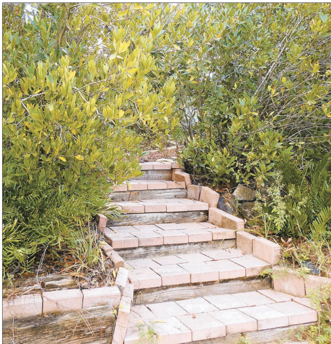
Colored concrete pavers make the treads of rustic steps while old pieces of pressure-treated lumber act as risers. At the top a path of crushed red bricks leads through dense evergreen native trees, shrubs and wildflowers. Passersby cannot see through to the home and front greenspace firebreak that surrounds it.
