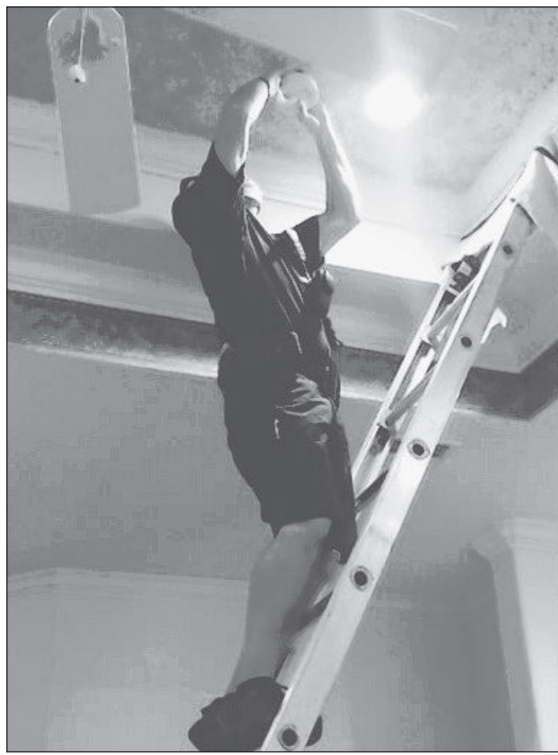
A Citrus County Fire Rescue staffer installs a smoke detector in a Citrus home.
