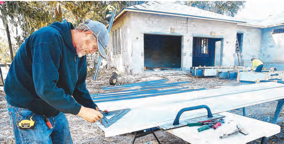
Certified Roofing Solutions, LLC foreman Mike Mizelle prepares to cut this steel panel Wednesday, March 10, that will be secured to the roof of a home in Crystal River.
